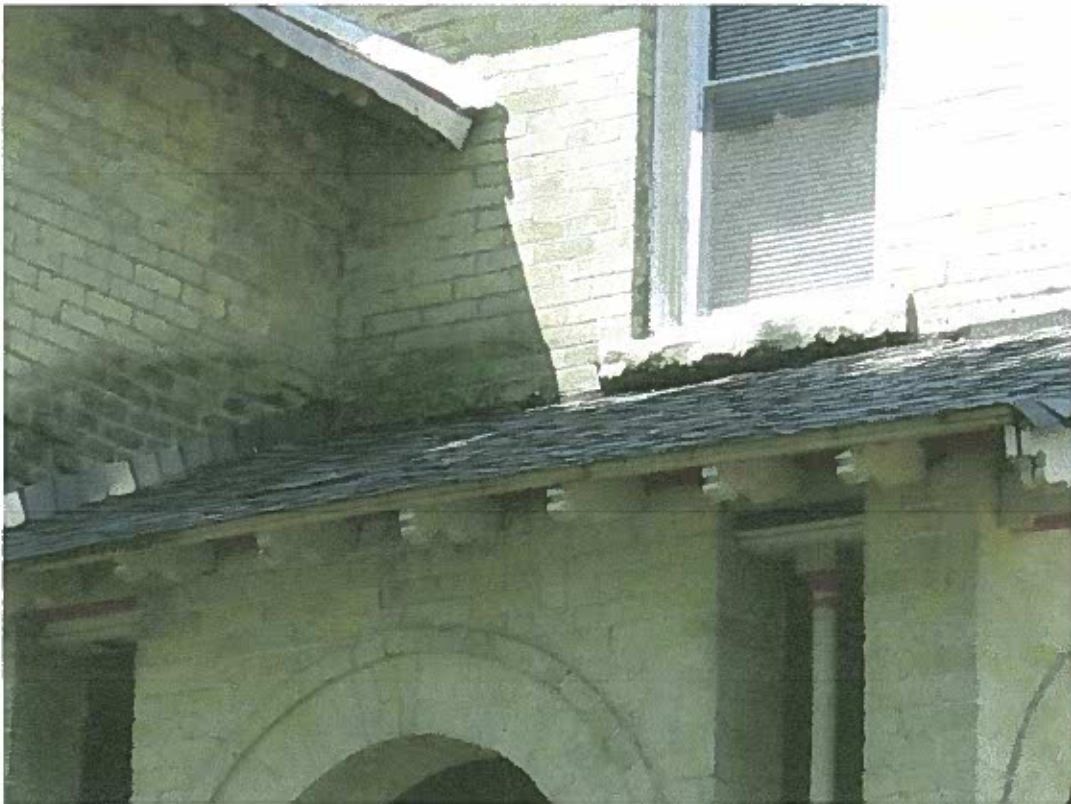
4. Closer view of the north east porch roof
