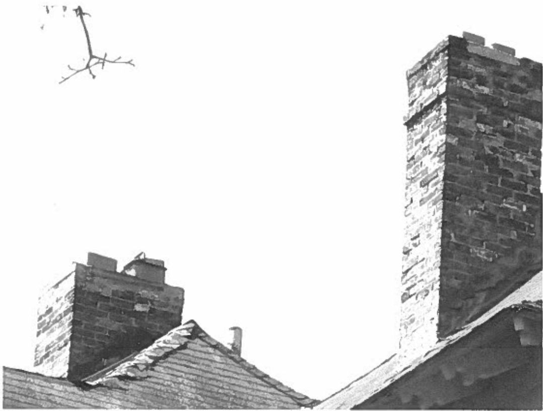
7. Close up of roof and chimney connections.
