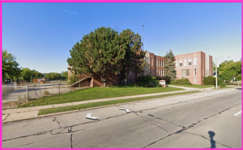
View from Silver Spring looking northeast
