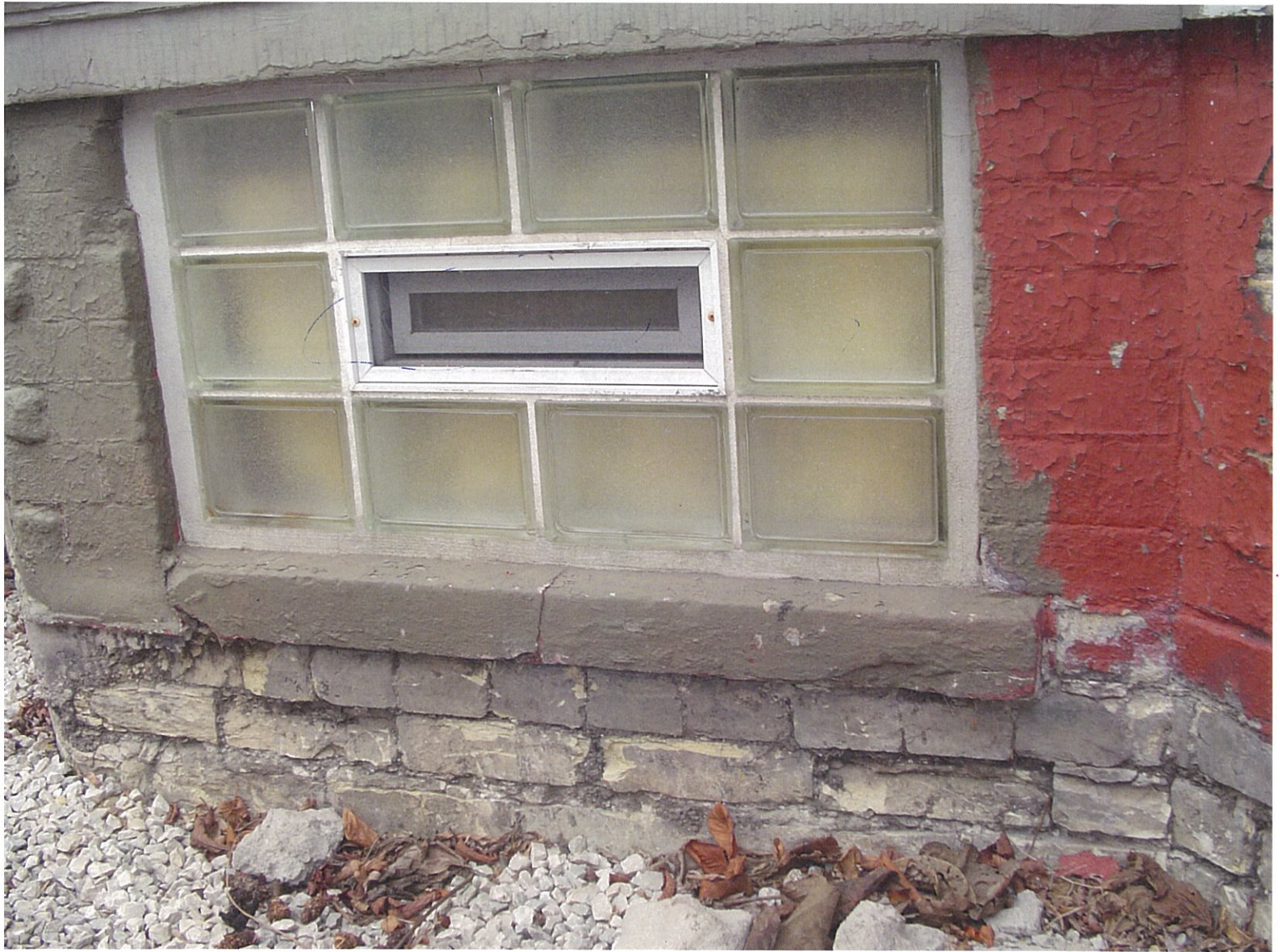
EAST BASEMENT GLASS BLOCK
