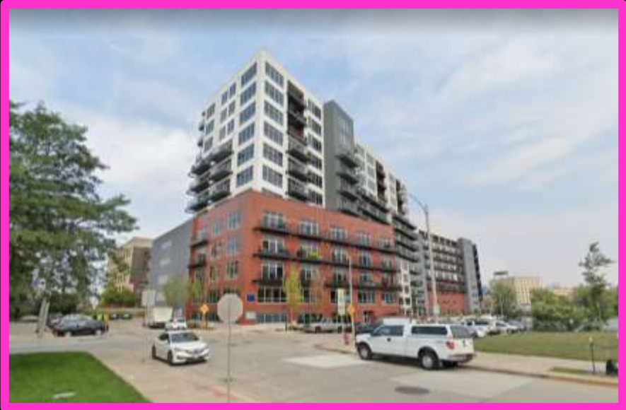
View from South 1 st St looking northwest
