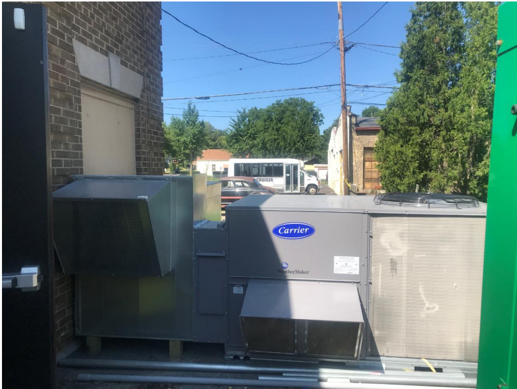
Photographs of the newly installed HVAC equipment at the northwest corner of the property, to be concealed by 6' wood privacy fence
