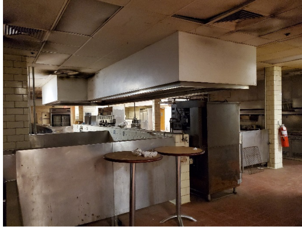
Photo 13: Kitchen on ground level in Building A.
