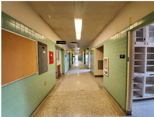
Photo 15: Corridor on top floor of Building A.
