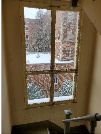
Photo 17: Stairway in Building A.
