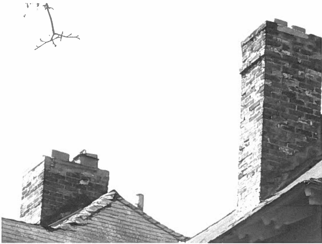
7. Close up of roof and chimney connections.
