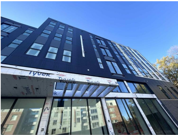
Siding on east elevation of north leg
