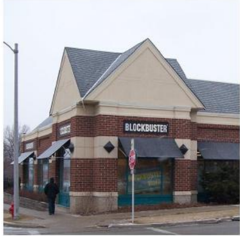
Image shows the existing corner condition.
