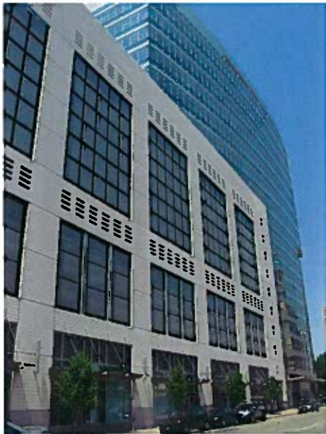
Example of well-designed parking structure facade and activated first floor at Cathedral Place on N. Jackson St. and E. Mason St.
