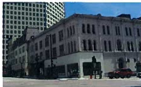
The Noonan Block building on East Wisconsin Ave. at Broadway
