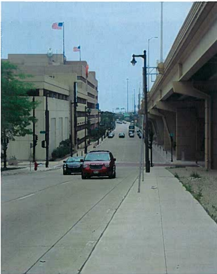
West Clybourn St. looking west from N. 6th St. is an example of a Type 4 Street
