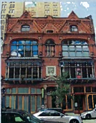
Building on Milwaukee St. between E. Wells St. and E. Wisconsin Ave.
