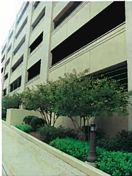
Parking garage with landscape edge
