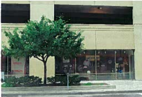
Hilton parking garage with first floor display windows engage the pedestrian
