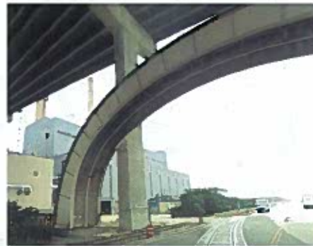
WeEnergies power plant in the Menomonee Valley on W. Canal Street distributes waste steam to Downtown for heating of buildings
