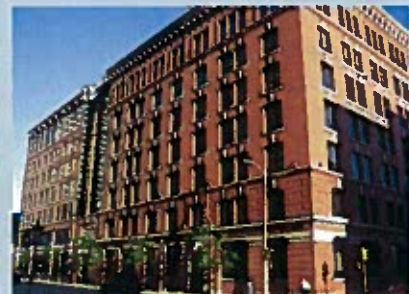
Johnson Controls, Inc. building on E. Michigan St. between N. Jefferson St. and N. Jackson St.
