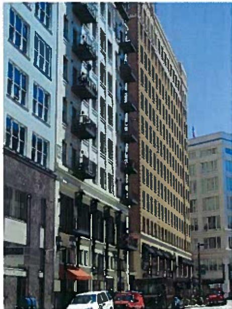
North Plankinton Ave. between W. Wells St. and W. Wisconsin Ave. looking south
