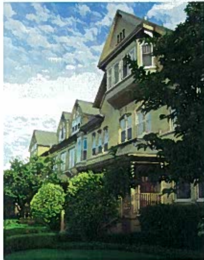
Rowhouses on E. Ogden Ave.
