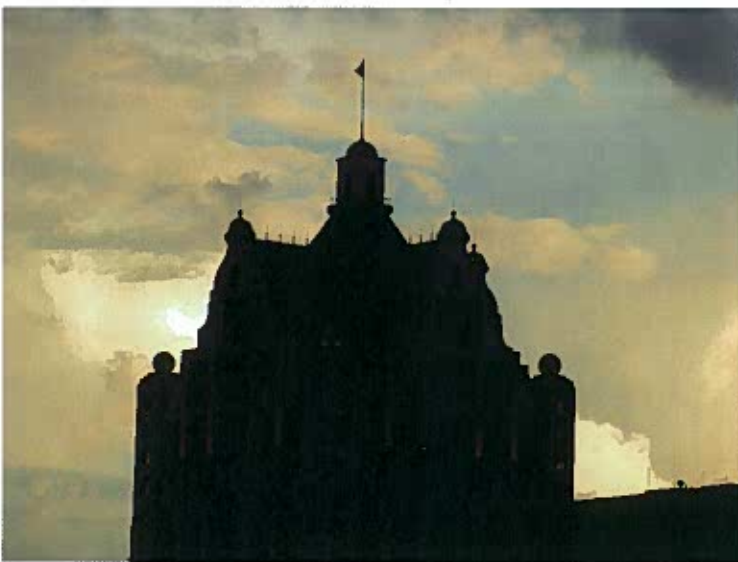
Articulated top of 100 East Wisconsin building at N Water St. and E. Wisconsin Ave.
