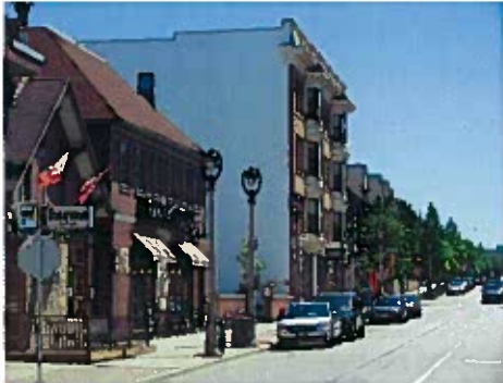
East Ogden Ave. looking east from N. Jackson St. is an example of a good Type 2 Street.
