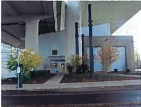
Streetcar maintenance facility under elevated freeway. Portland, OR
