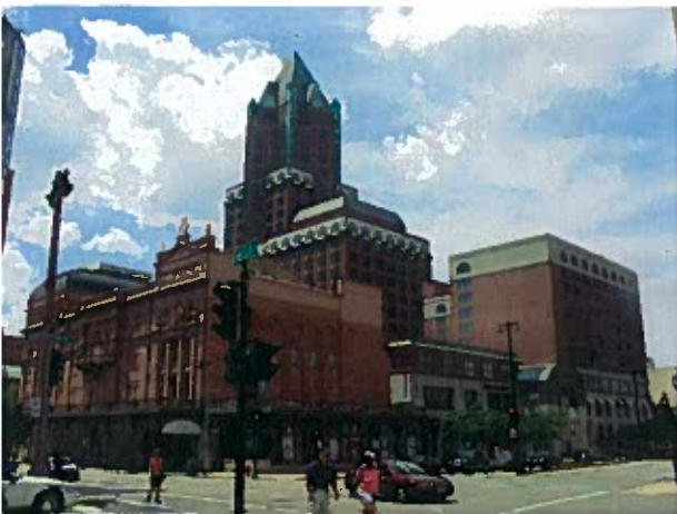
The Milwaukee Center on N. Water St. and E. Kilbourn Ave. integrated several historic structures into its development which contains theaters, hotel, offices
