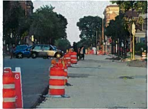
East State Street under reconstruction, a conversion to two-way circulation
