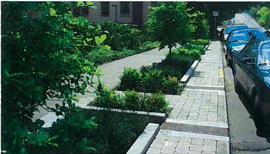
Stormwater retention integrated into streetscaping pattern on a residential street in San Mateo County, Ca
