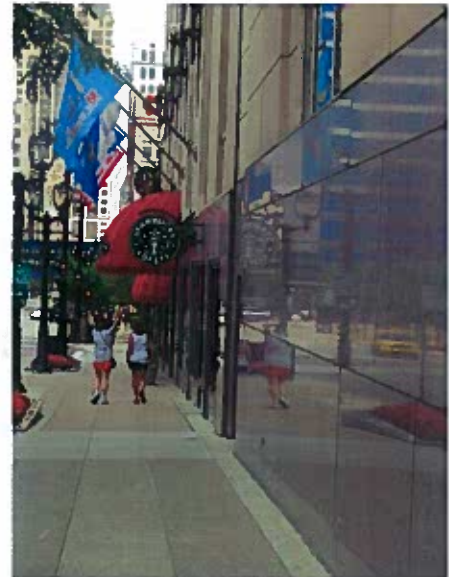
Hilton Hotel facade wall with high quality granite cladding
