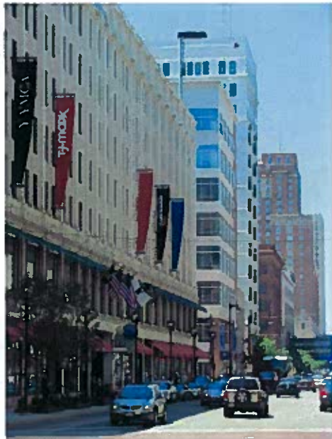
UW-Milwaukee and the YMCA occupy space in the Grand Avenue complex
