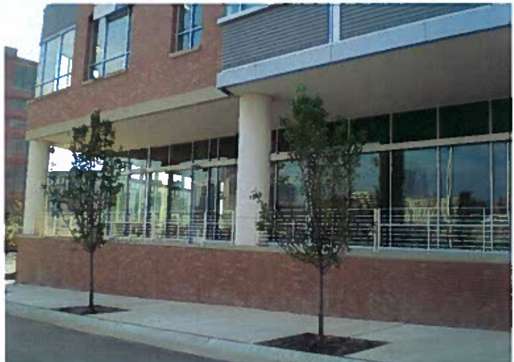
Streetfront cafeteria windows and outdoor area at Manpower World Headquarters facing the Milwaukee River
