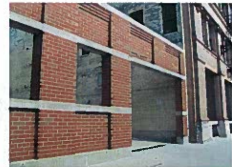
A masonry wall fills out the street edge
