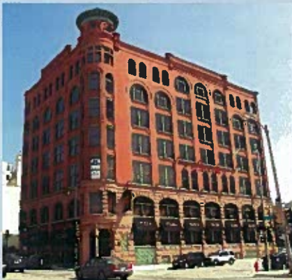
Button Block building at N. Water and E. Clybourn Streets
