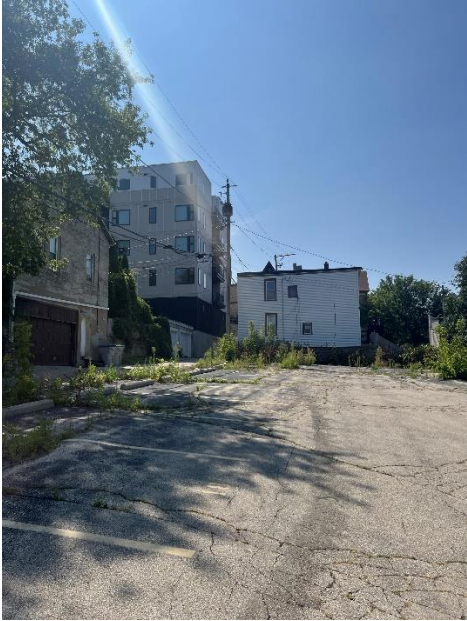
Existing parking lot along existing alley. View looking south.
