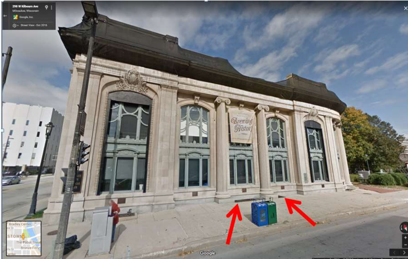
Kilbourn façade with wells to be capped indicated by arrows.
