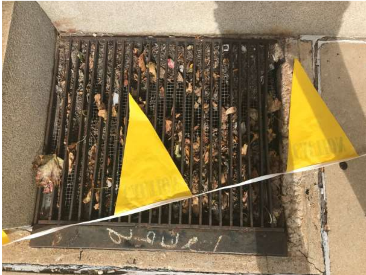
Current state of smaller (east) well, looking north.
