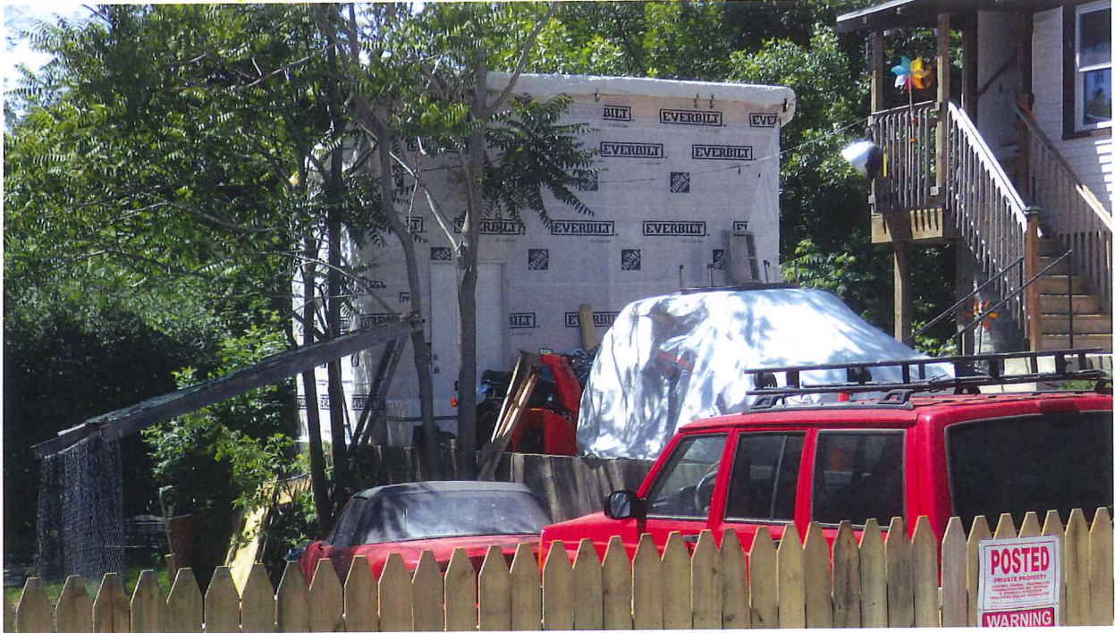
3217 N 5th Street. 6/21/2022. (G. Armstrong/ Special Enforcement) (Violation # 1. Outdoor Storage Facility).
