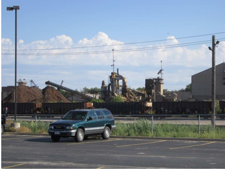
South View from Biogas Generation Site
