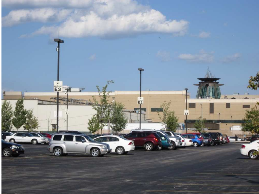
East – Northeast View from Biogas Generation Site
