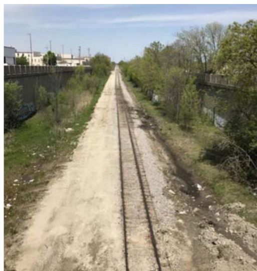
30 th St. Rail Corridor
