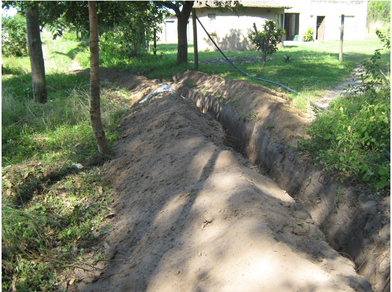
The trench has been dug using a labour intensive methods
