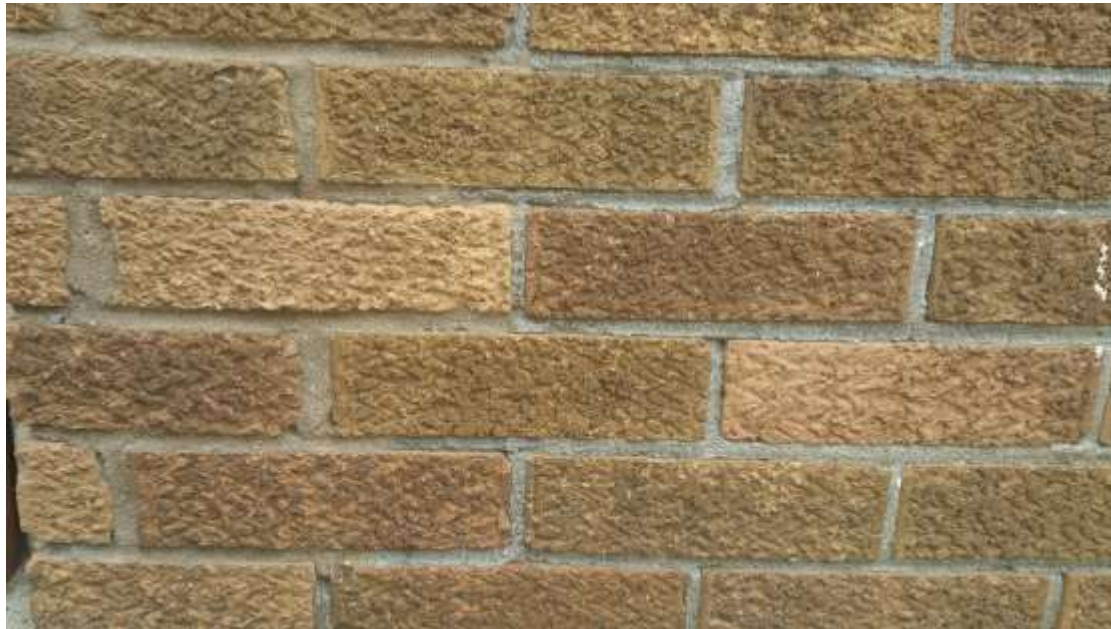
Detail of original brick
