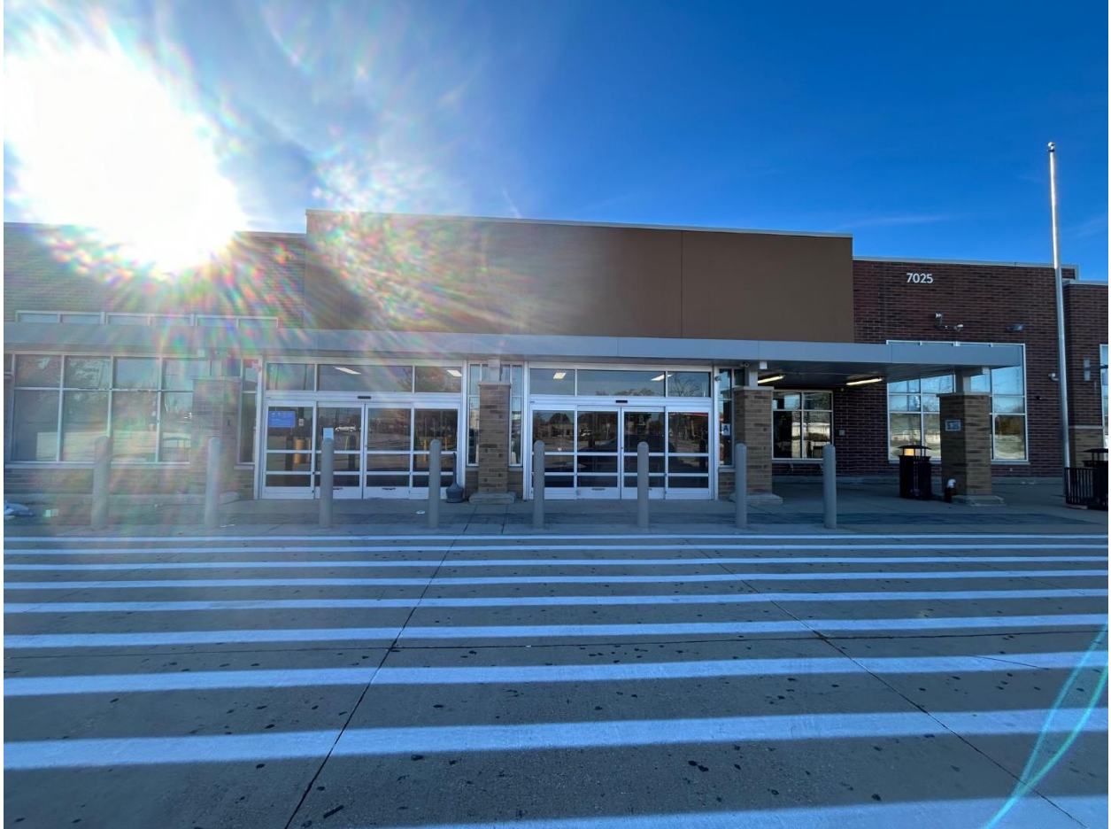
Store Main Entrance
