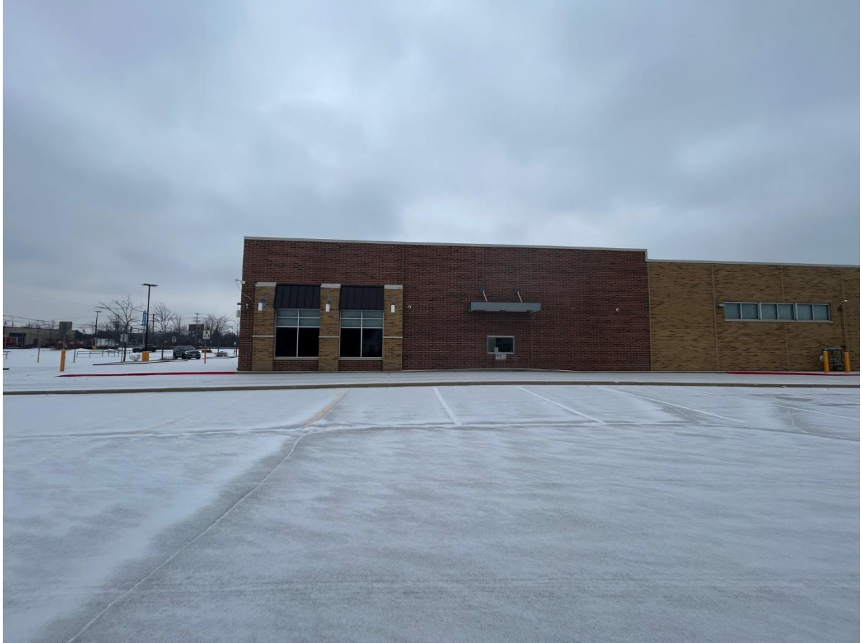
Additional parking and north side of store
