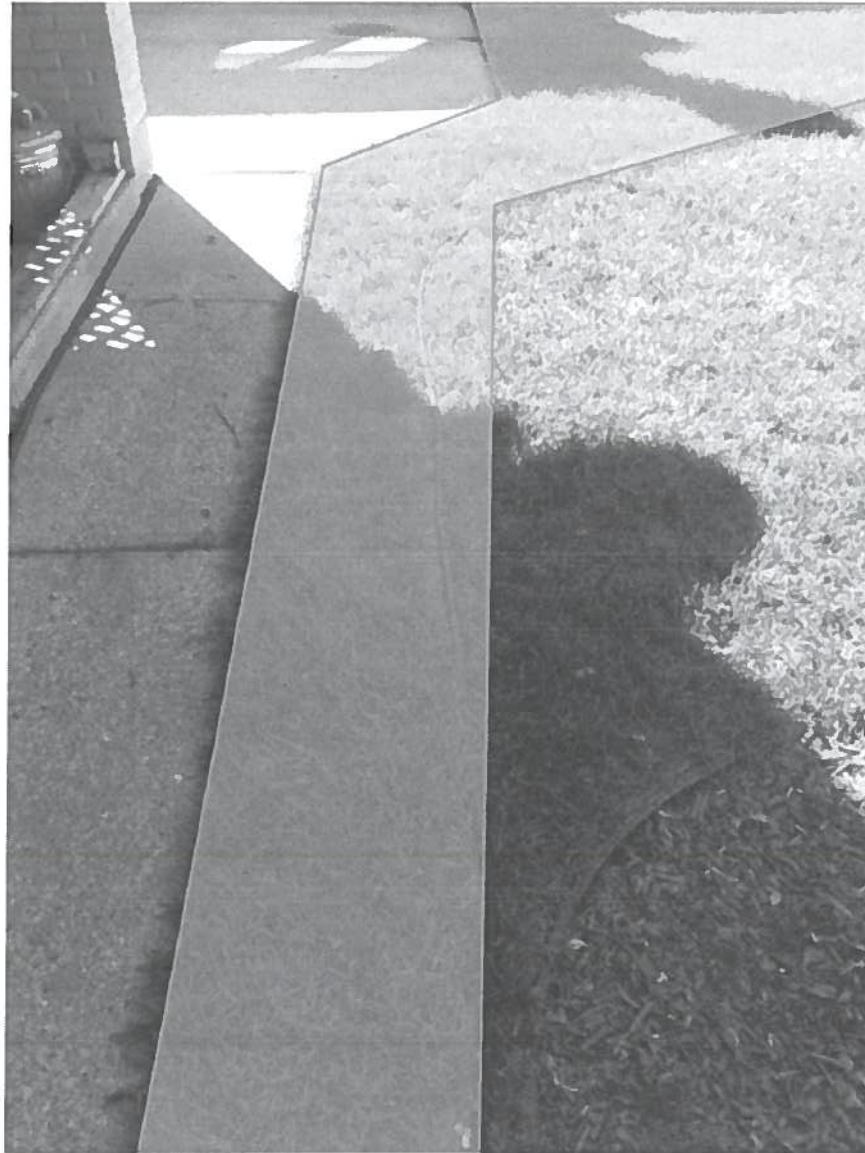
Addition to current rear sidewalk.
