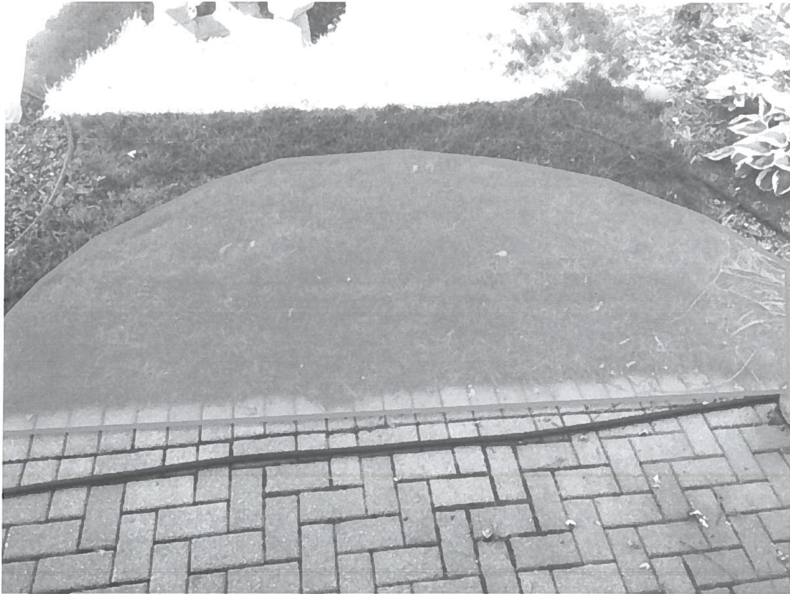
Replace rear pavers and expand with poured concrete.
