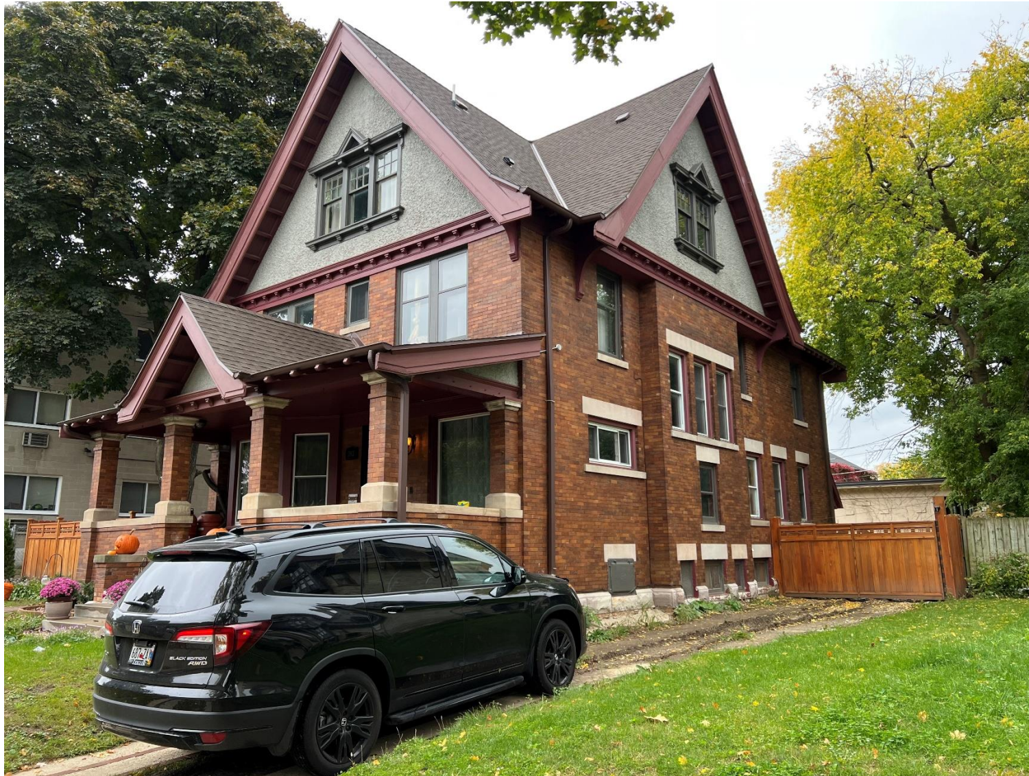
Driveway to be poured in line with current location
