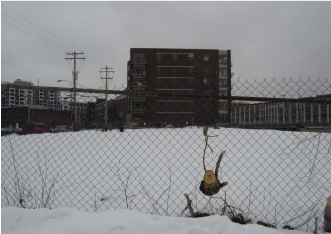
236 S. Water Street-West View
