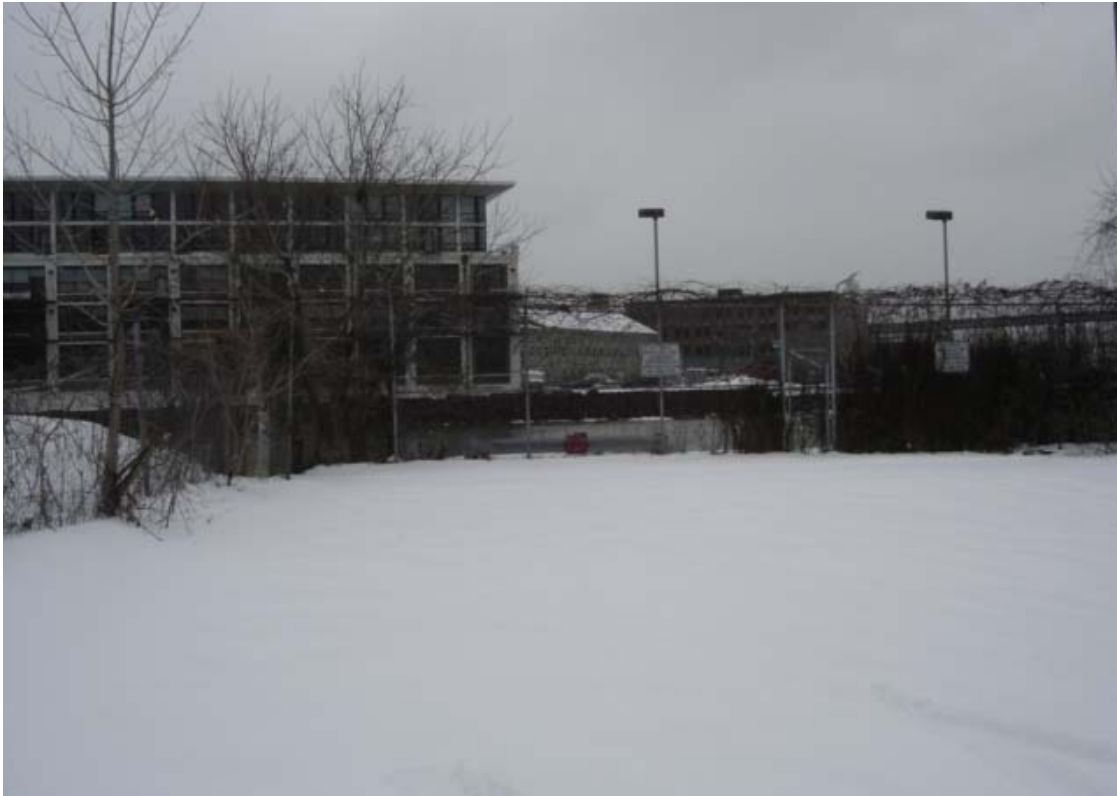
236 S. Water Street- View Across River to North
