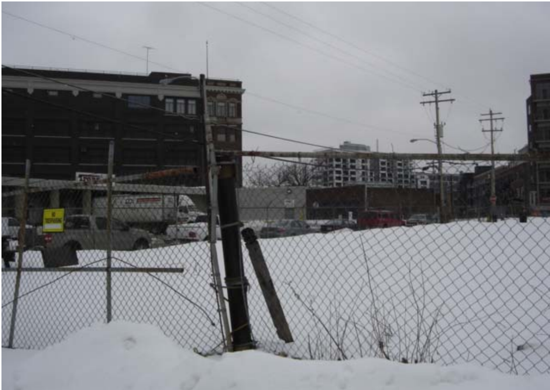
236 S. Water Street-South West View
