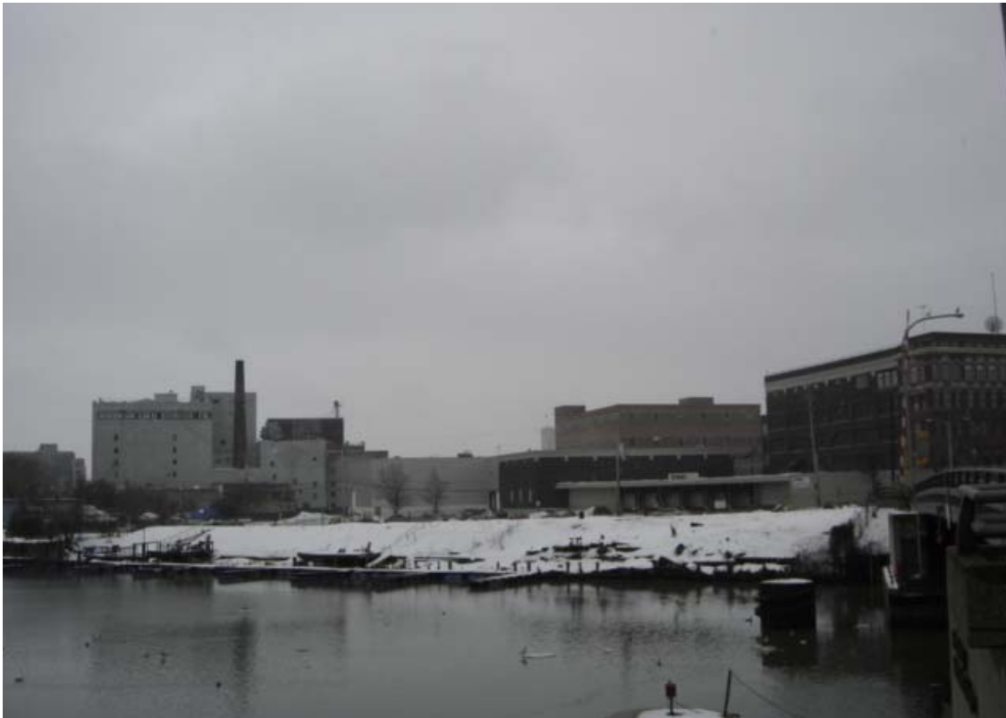
Pittsburg Avenue on Bridge-View South
