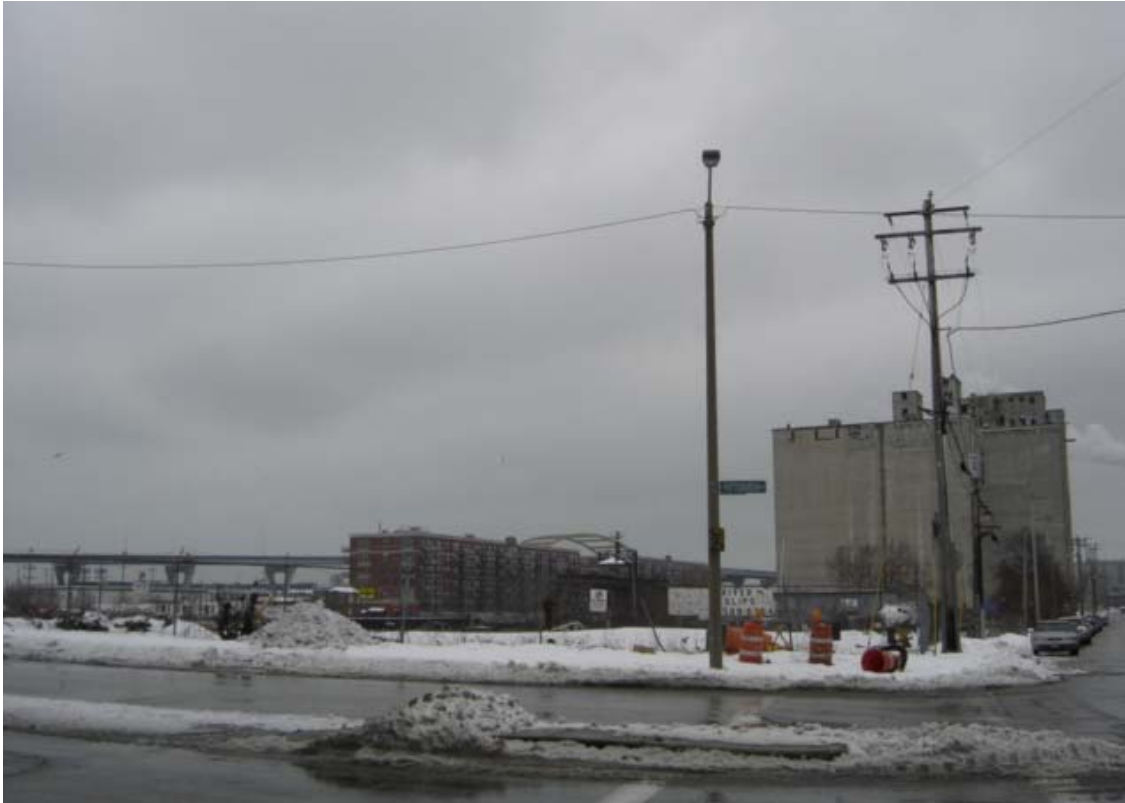
Corner of Water Street and Pittsburg-East view
