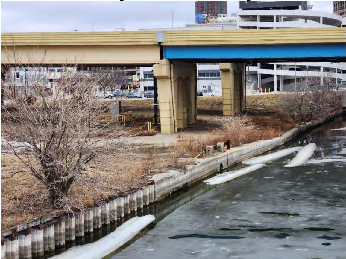
Location where alley, Riverwalk (trail) and the two projects meet Looking north from St. Paul Ave. bridge
