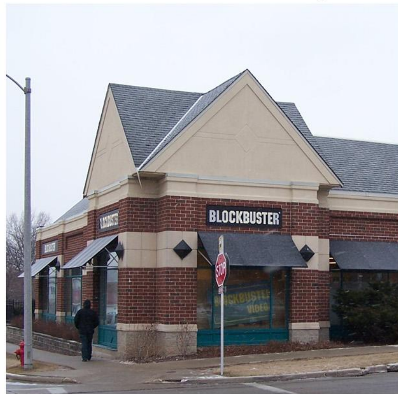
Image shows the existing corner condition.
