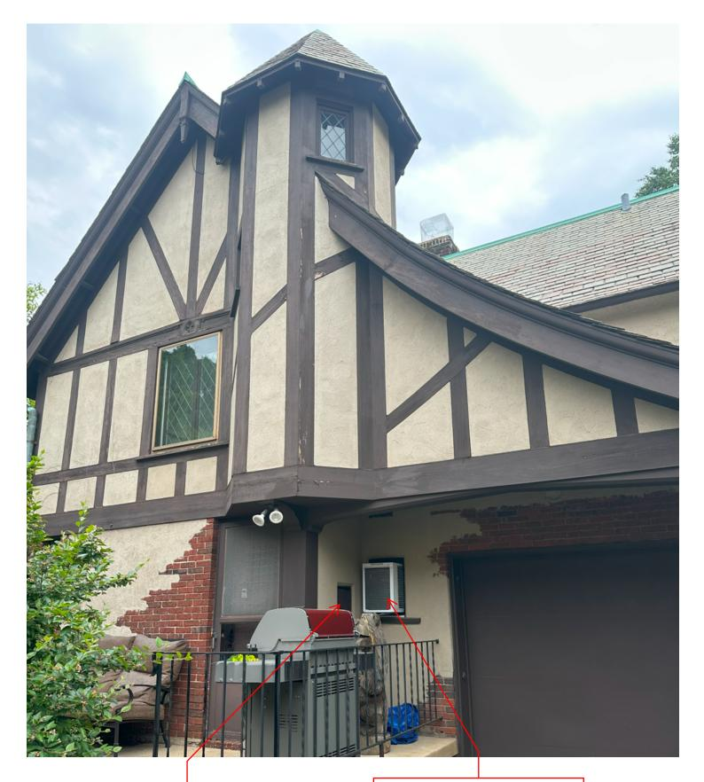
HISTORIC MILK DELIVERY DOOR REMAINS. AC UNIT TO BE REMOVED FROM WINDOW OPENING AND REPLACED WITH MARVIN ULTIMATE WINDOW. SEE NEXT PAGE FOR WINDOW SPEC.
