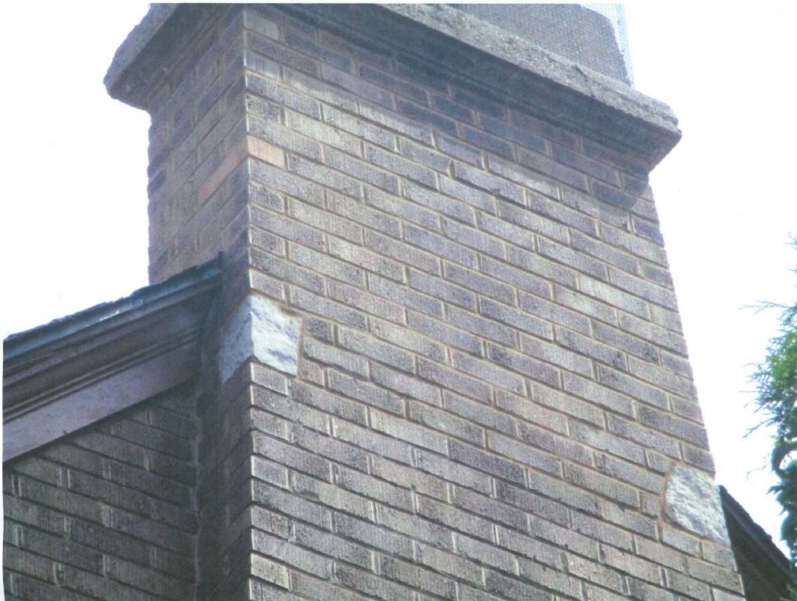
Chimney as repaired
