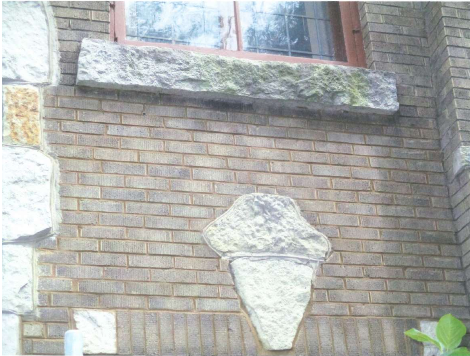
Repairs between first and second floors
