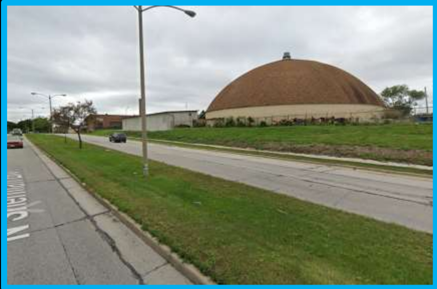
View from North Sherman Blvd looking south-west
