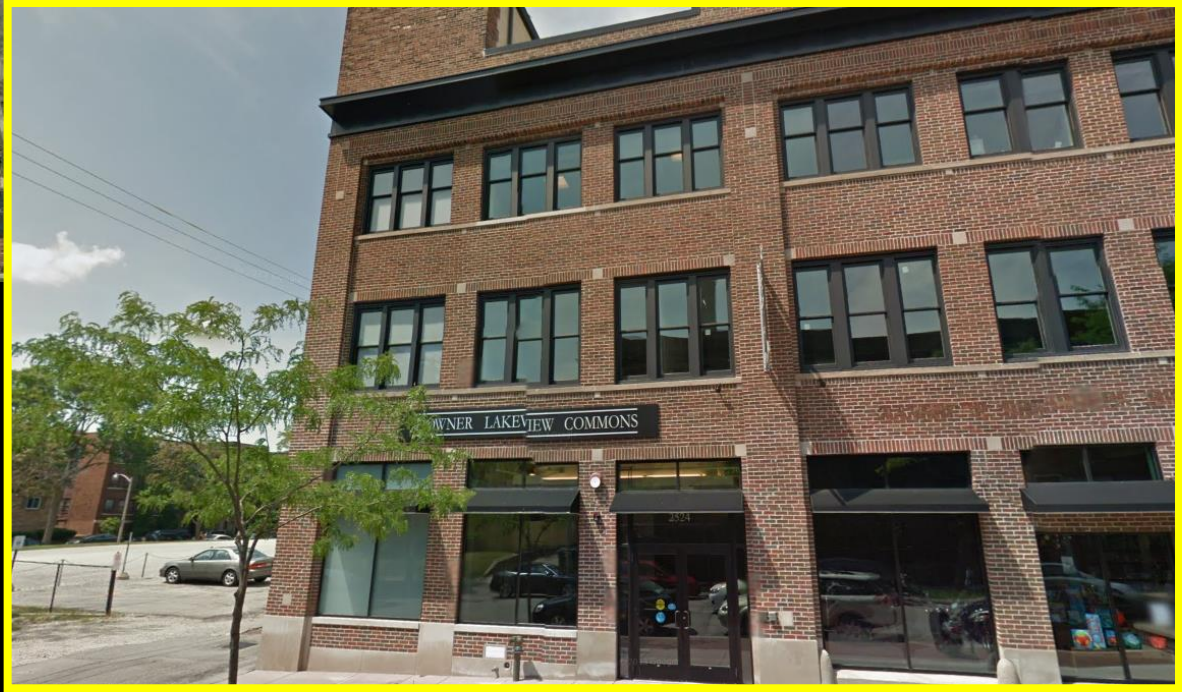
View of building from E Webster Pl, looking north
