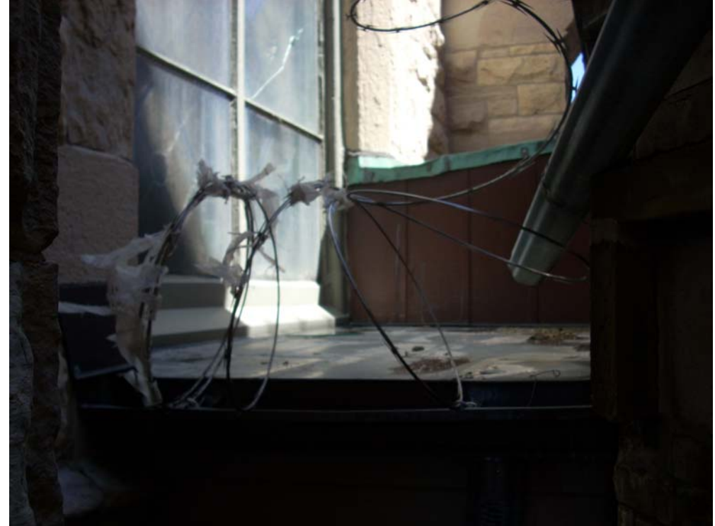
Existing roof at church window
