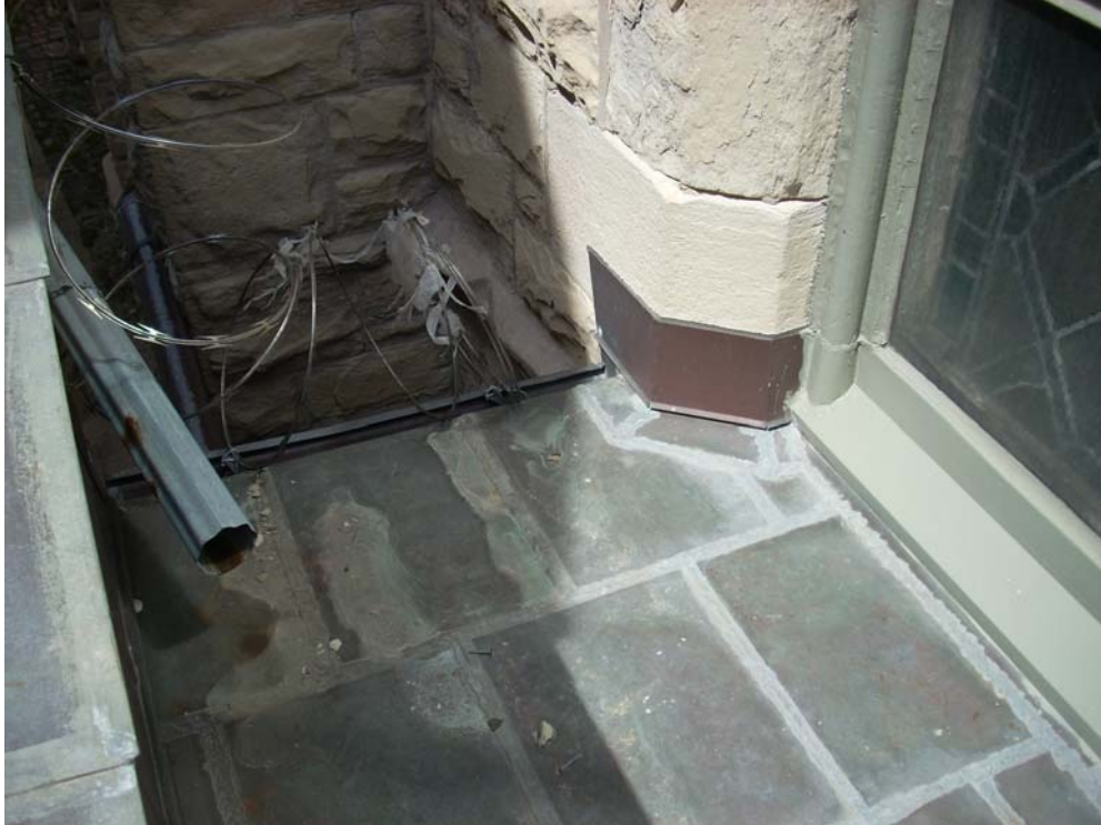
Existing roof at church window
