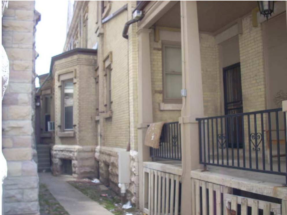
Existing rectory North elevation
