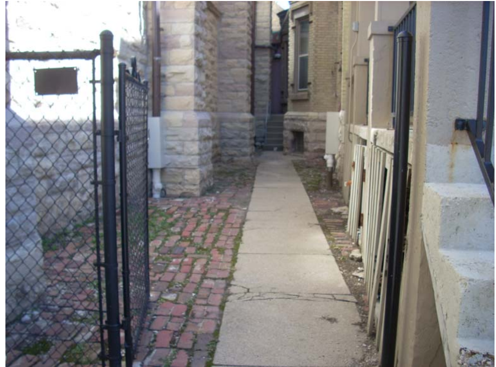
Existing conditions looking East
