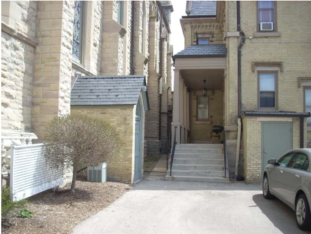
Existing conditions looking East
