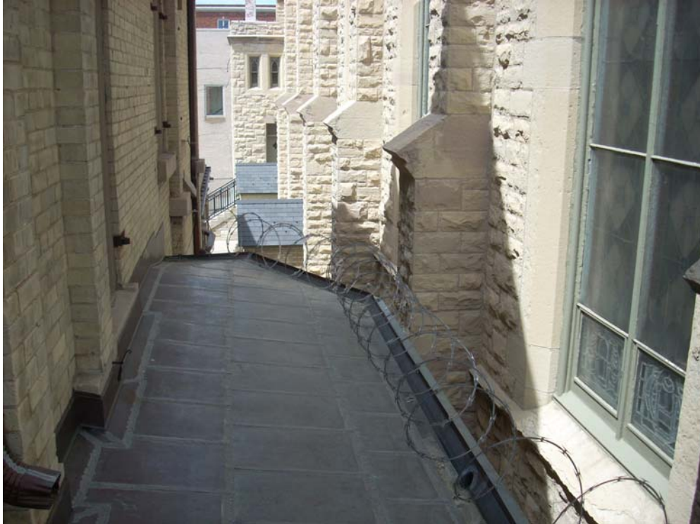
Existing rectory low roof
