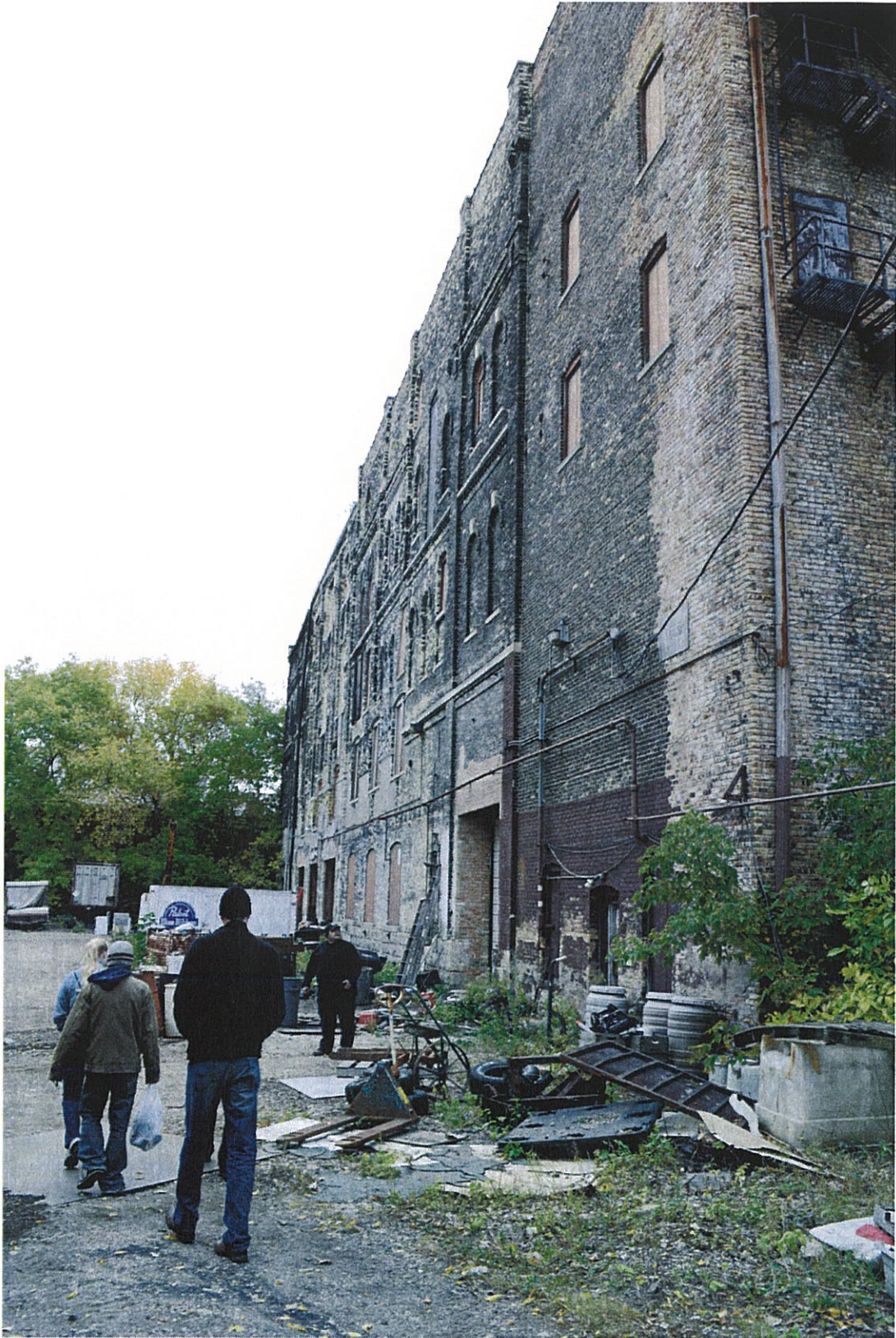
Longview perspective of northern façade of Brewery building.
