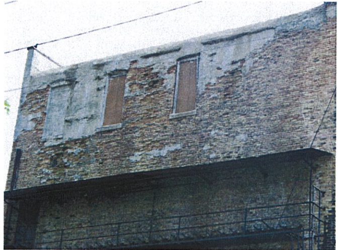
West facing façade with closeup of spalling brick wall.
