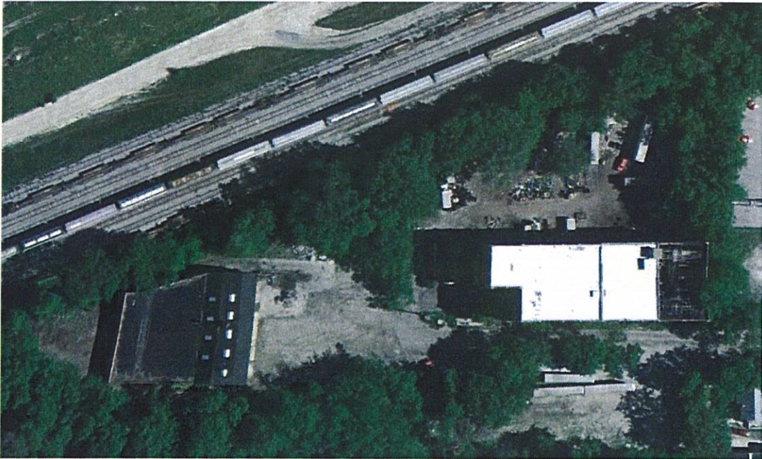
Overhead view of subject property. The “Stables” building is on the left, and the “Bank” and “Brewery” buildings are on the right. This photo clearly shows the collapsed roof area of the “Brewery” structure.
