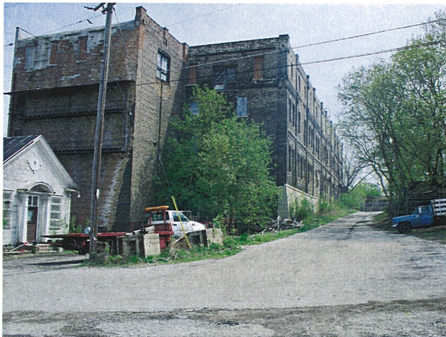
Southwest view of Brewery Building.
