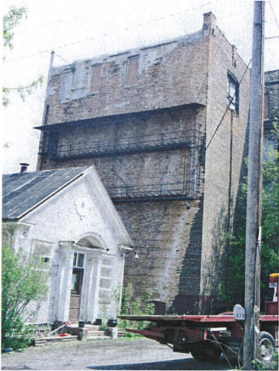
West facing façade with closeup of spalling brick wall.
