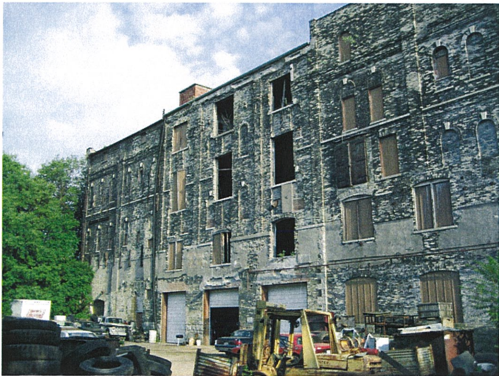
Northern façade of Brewery structure (cameraman is looking southeast).
