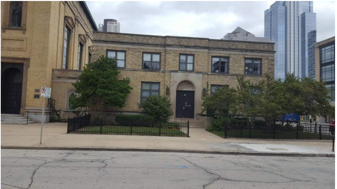
Exhibit B View of west facade along N. Jackson St. Ramp and stair are generally obscured by trees.
