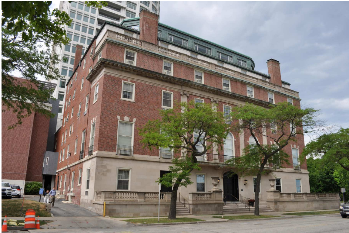
Photo 5 - View of Southwest Elevation of the University Club from across Wells Street
