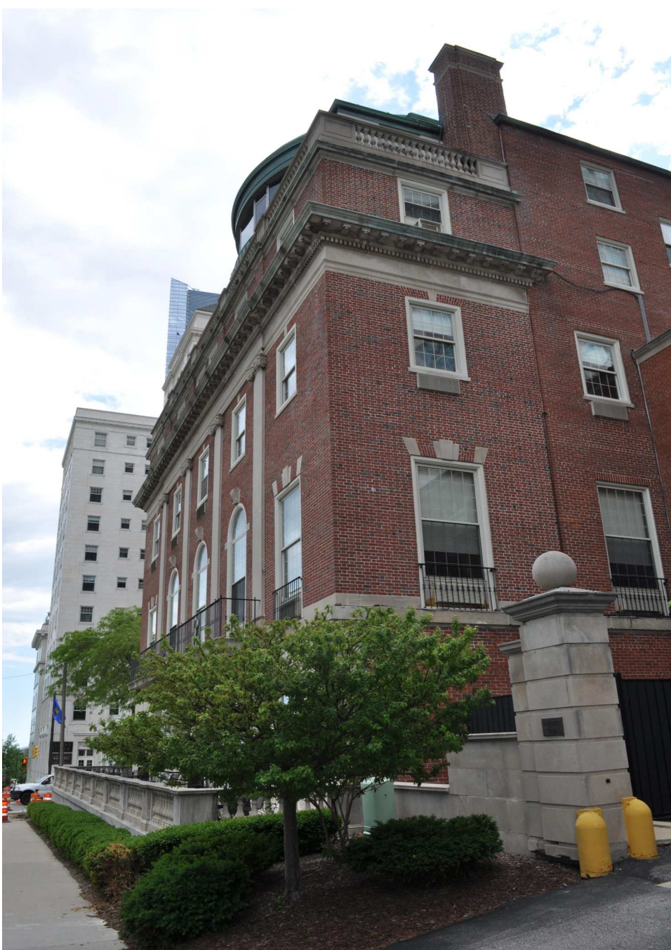
Photo 7 - View of North Elevation of the University Club from Sidewalk
