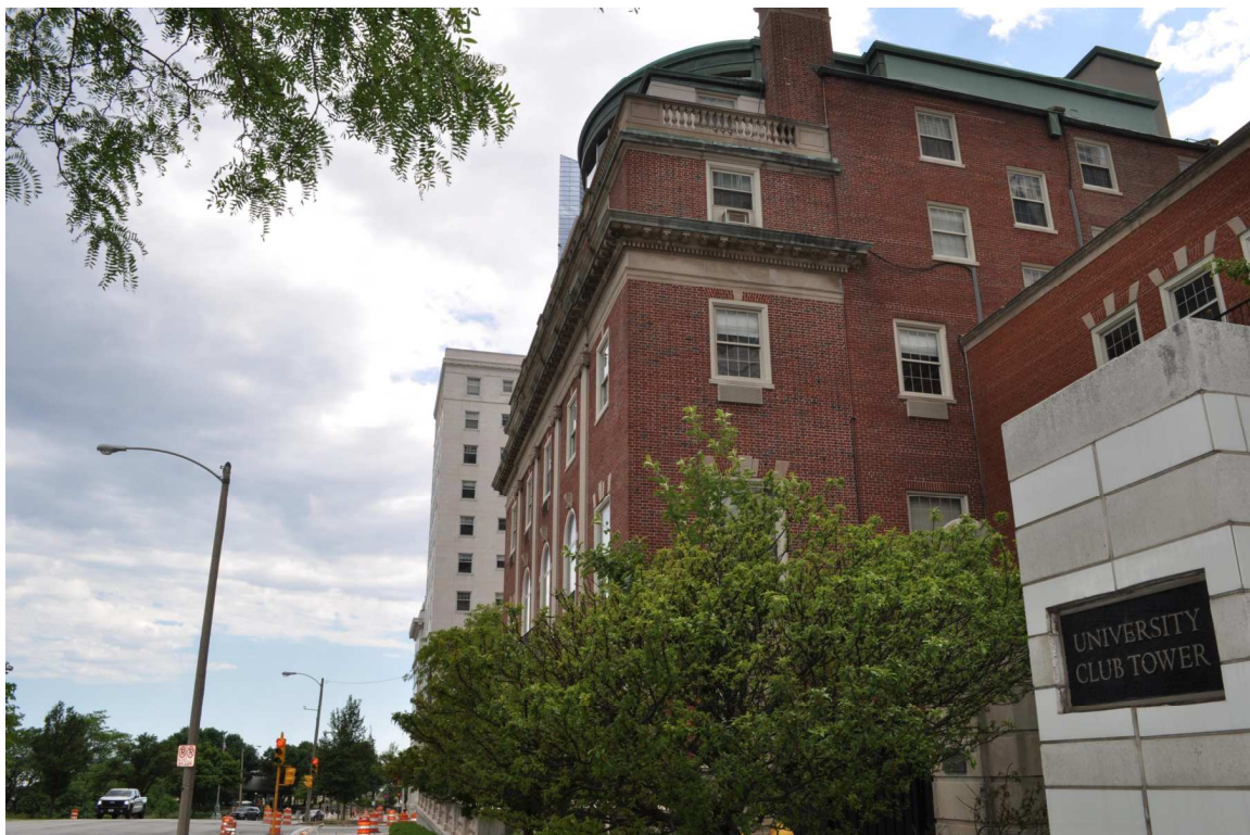
Photo 6 - View of North Elevation of the University Club from Sidewalk
