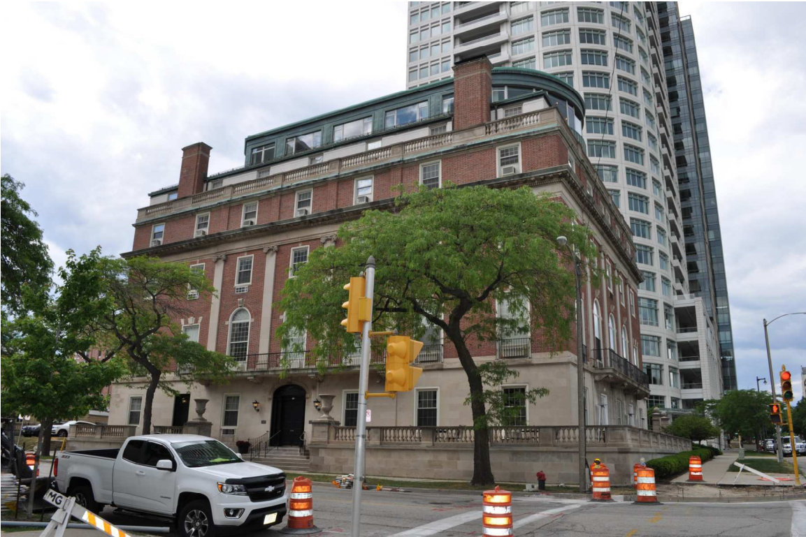
Photo 4 - View of Southeast Elevation of the University Club from across Wells Street
