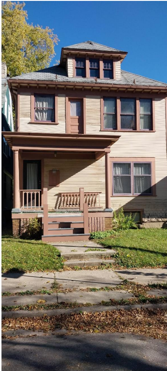
New stairs, posts, and railings on front steps
