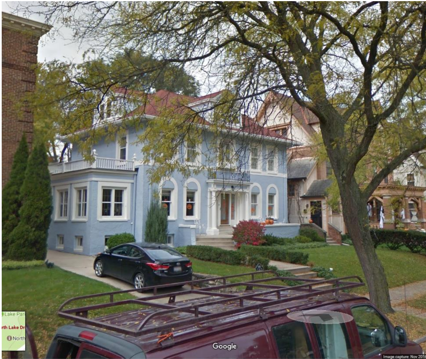
Present conditions at front of house.
