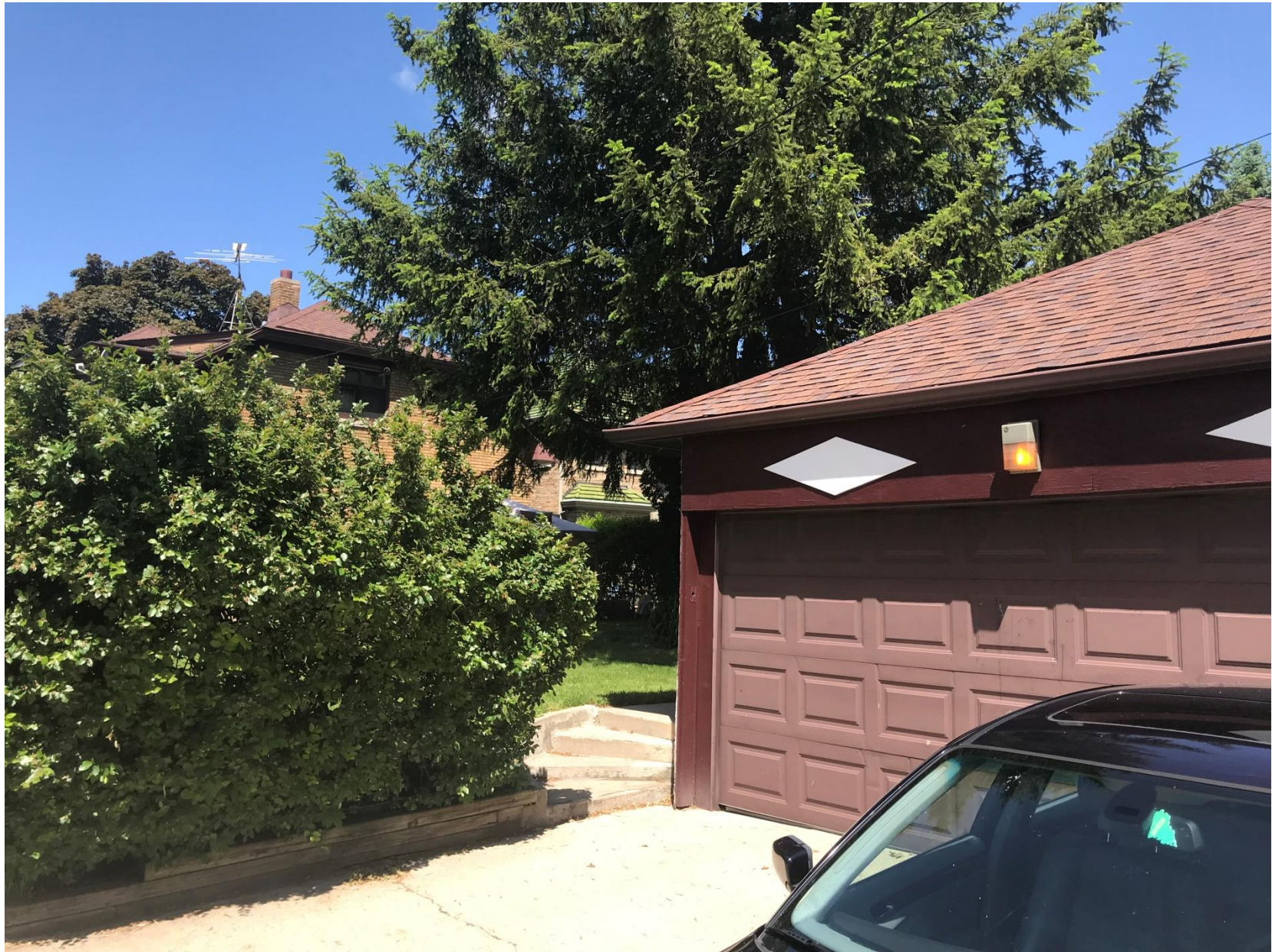
Gate to be installed at these steps down to the garage.
