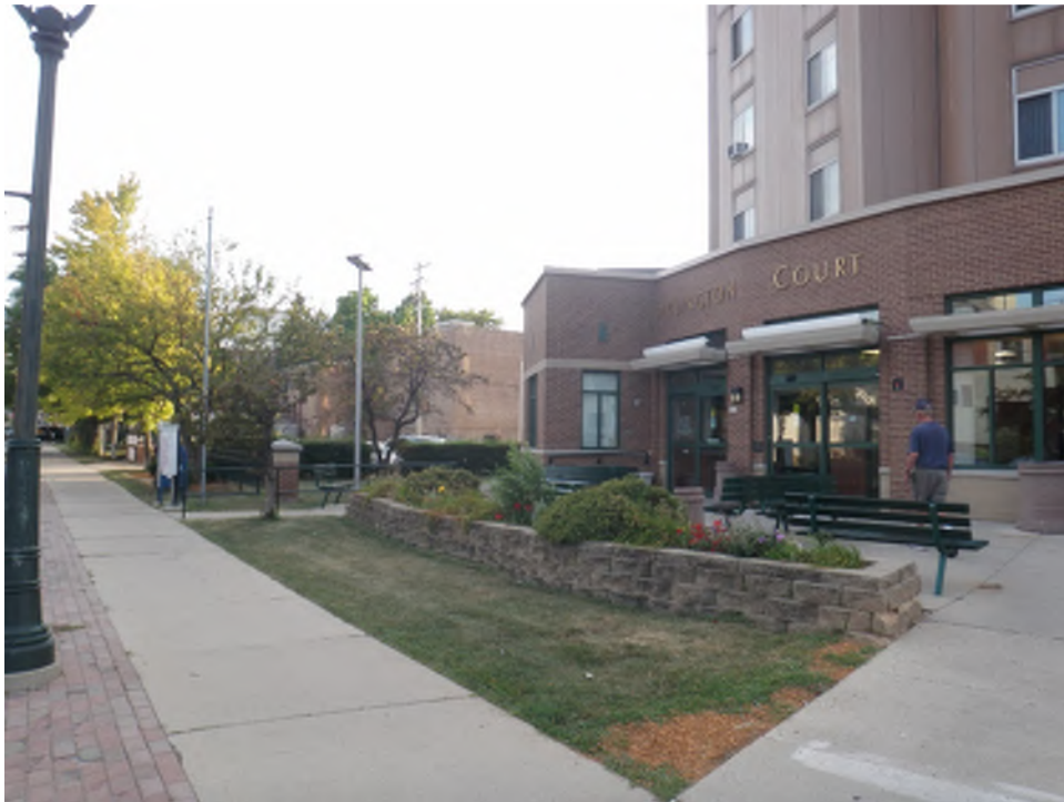
Photo 12 – View southwest on Arlington Place
