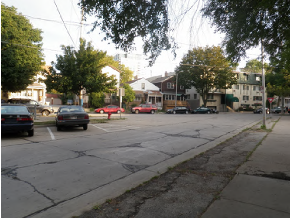
Photo 15 – View southeast on Arlington Place
