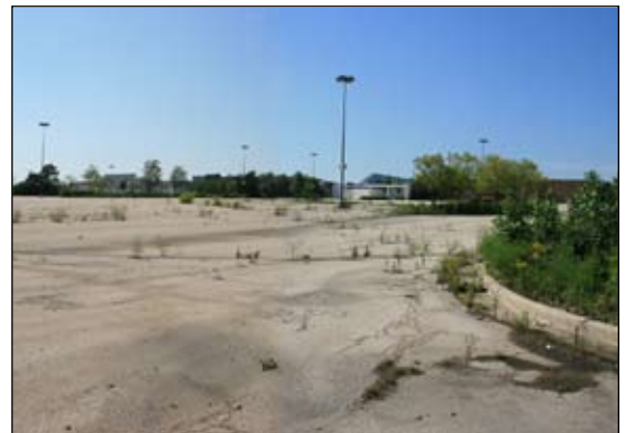
Existing conditions of the former Northridge Mall structure.
