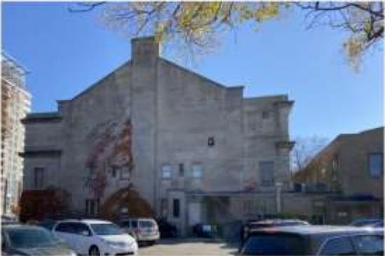
Existing 1451 N Prospect (Renaissance Place) - West Facade
