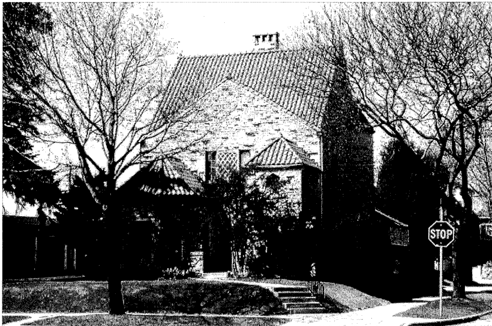
Vents to be located to rear of dwelling (preferable) or on rear of south elevation.
