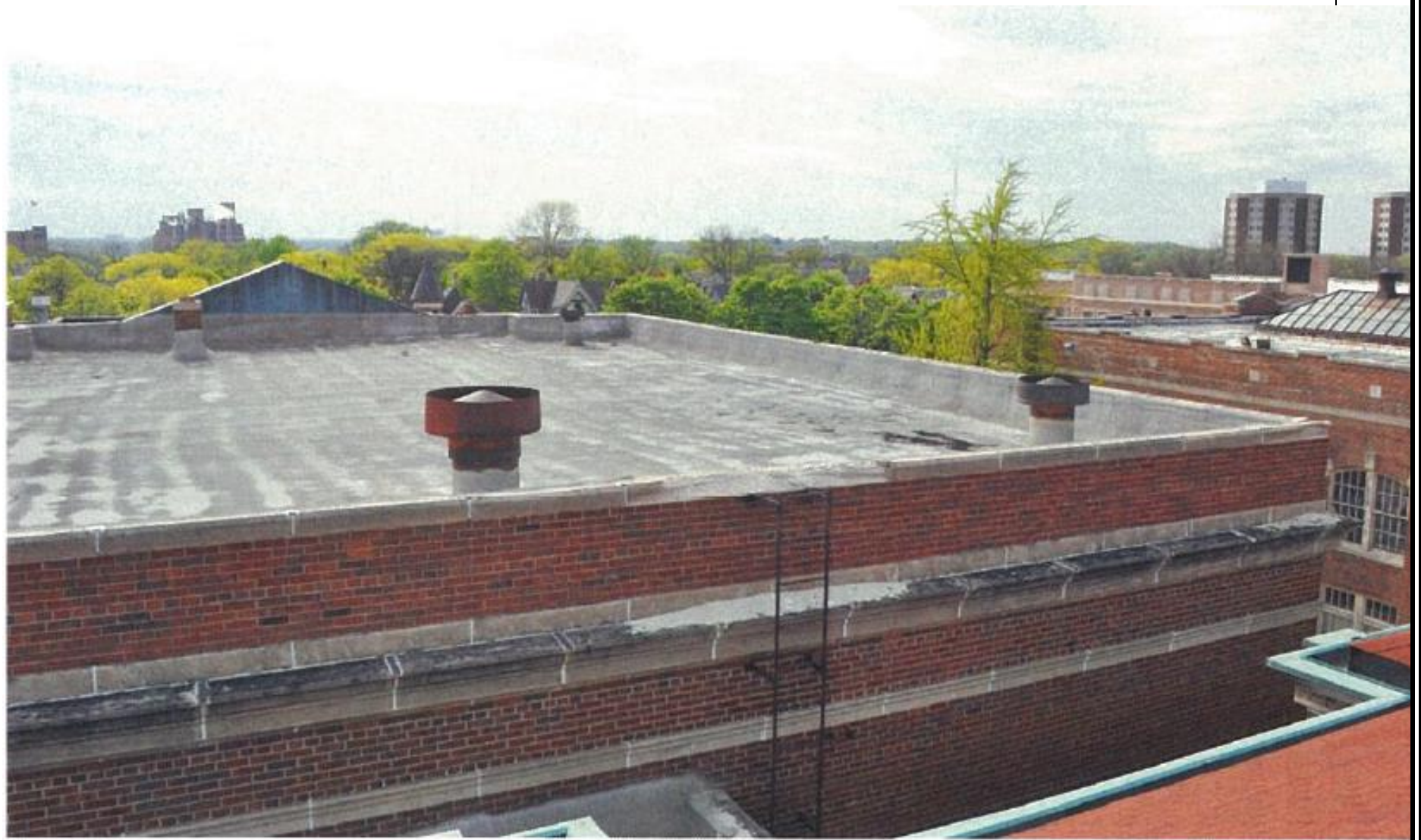
Photo 8 – Library Roof, looking northwest
