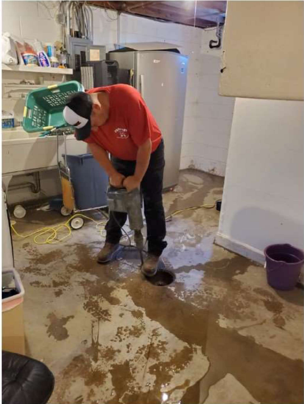
set 4: Palmer valve opened by Ever Dry 10/1/21
