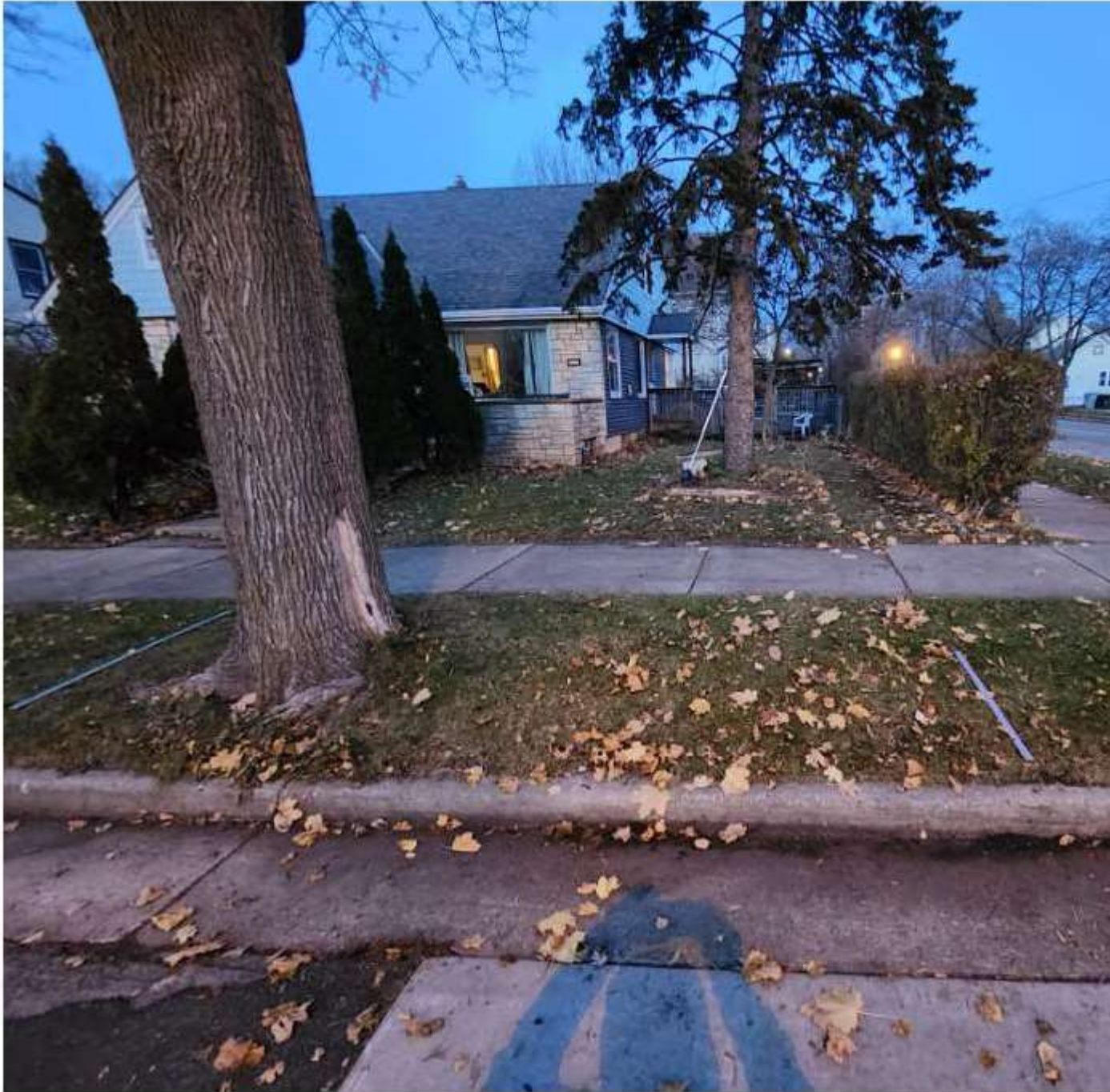
set 3 : metal yardstick on right shows about where leak was found in front of my house
