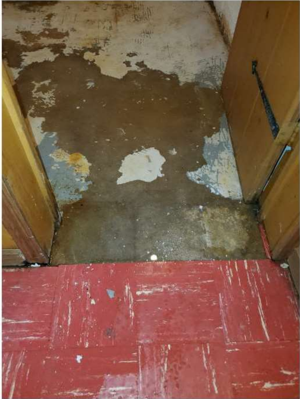
set 1; 9/22/23 entry to cellar
