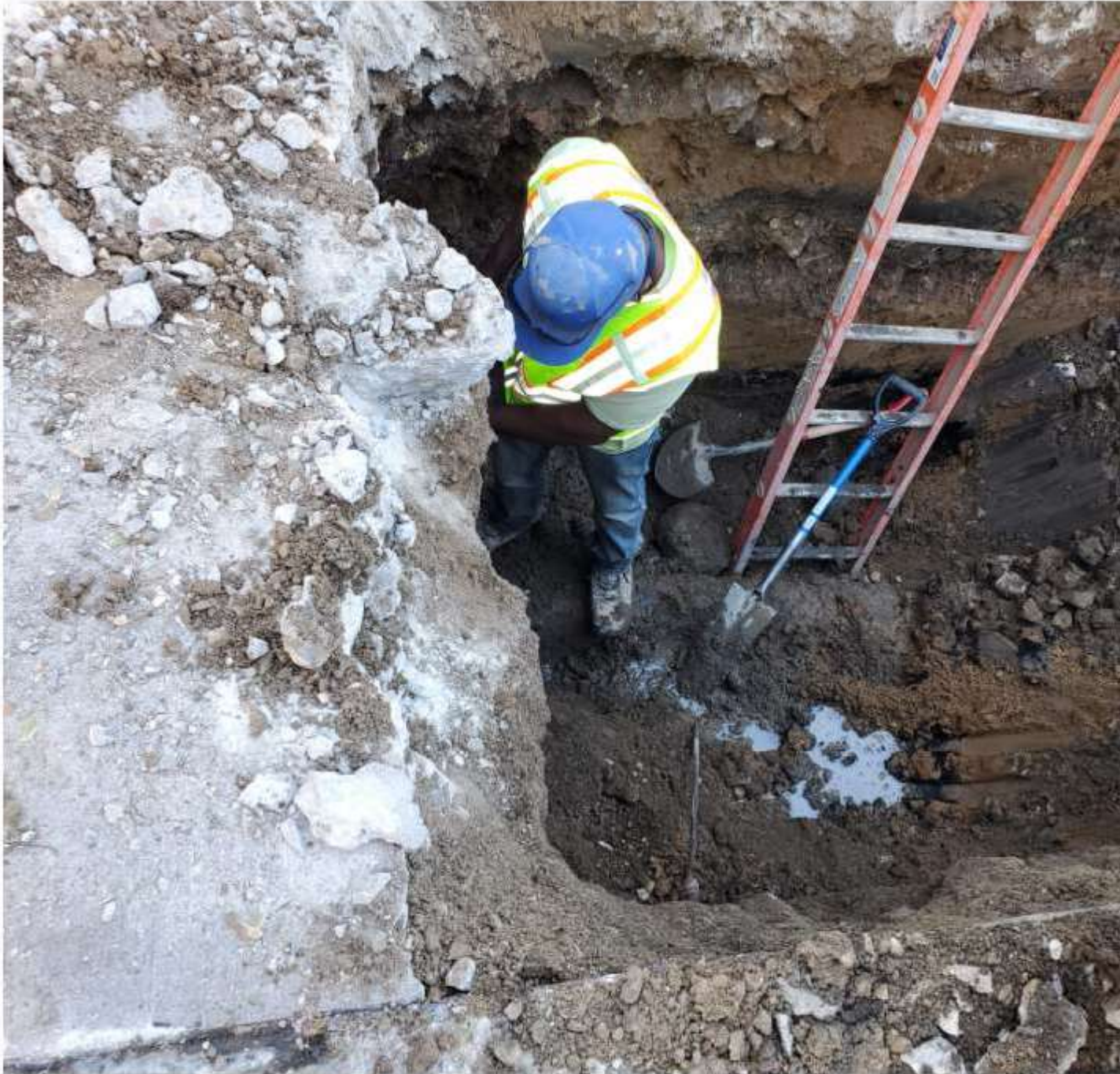
set 2: 9/30/21 1st dig near driveway, water starting in hole
