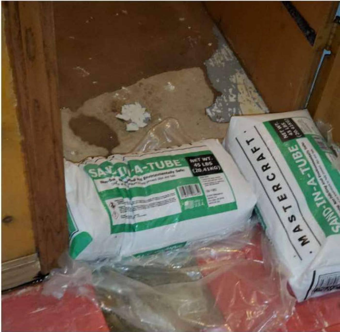
set 2: 9/26/21 sandbags to contain cellar water
