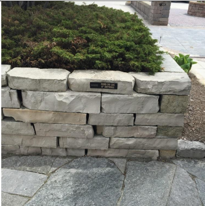
Retaining wall style in coursed rough-faced white stone
