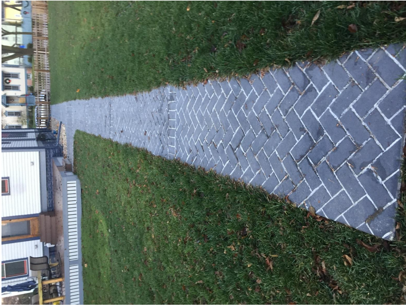
Pattern and color of stamped and stained concrete for extended walkway
