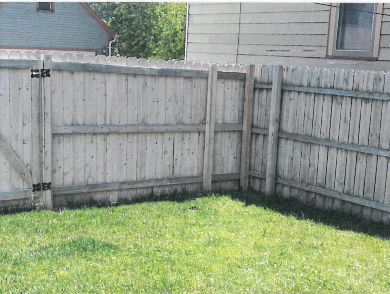
3 of 3 showing southeast corner of fence
