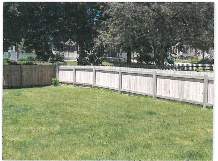
4 of 4, showing northwest corner
