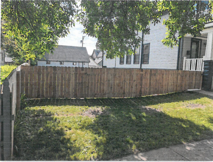
Street view of fence on north side of house
