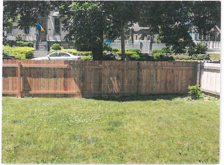
Reverse of fence facing street on north side of house. 2 of 2
