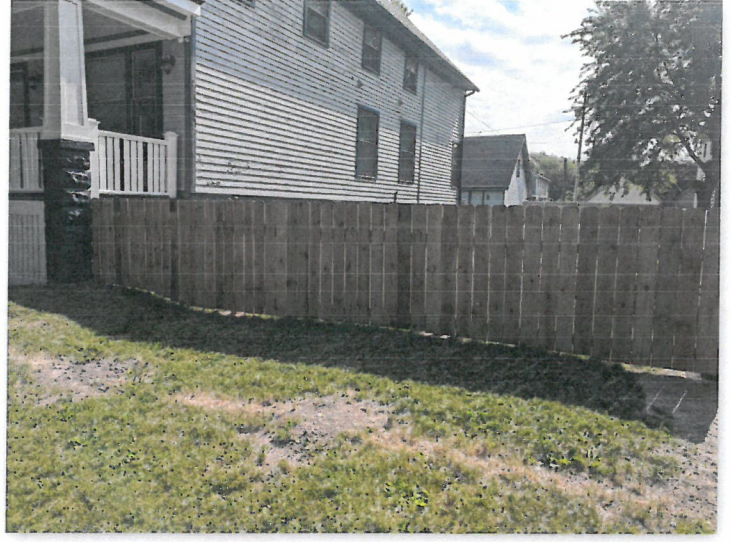
Street view of fence on south side of house
