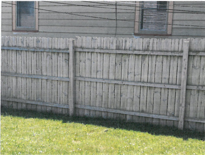
3 of 6, showing reverse of south side fence.
