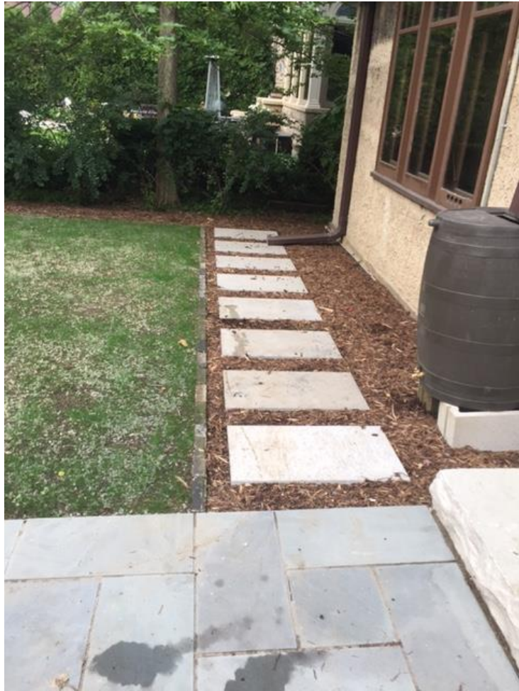
Partially completed work, new pavers and limestone step.
