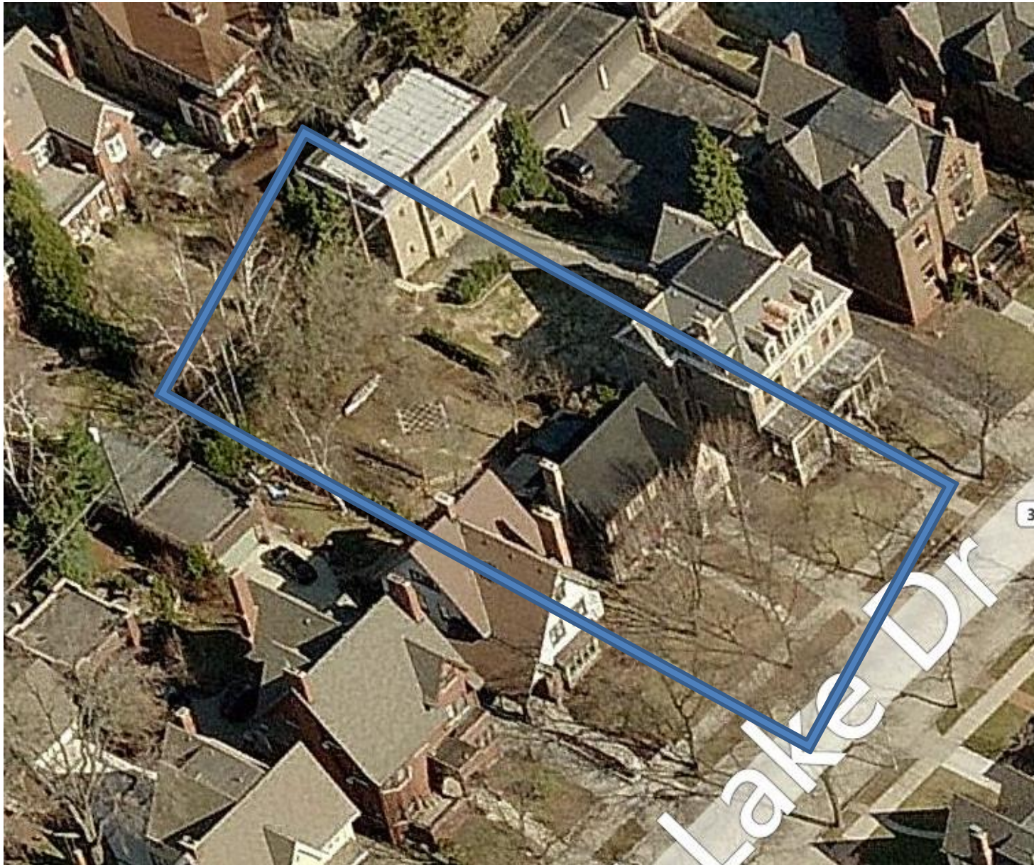
Aerial view of property prior to work.
