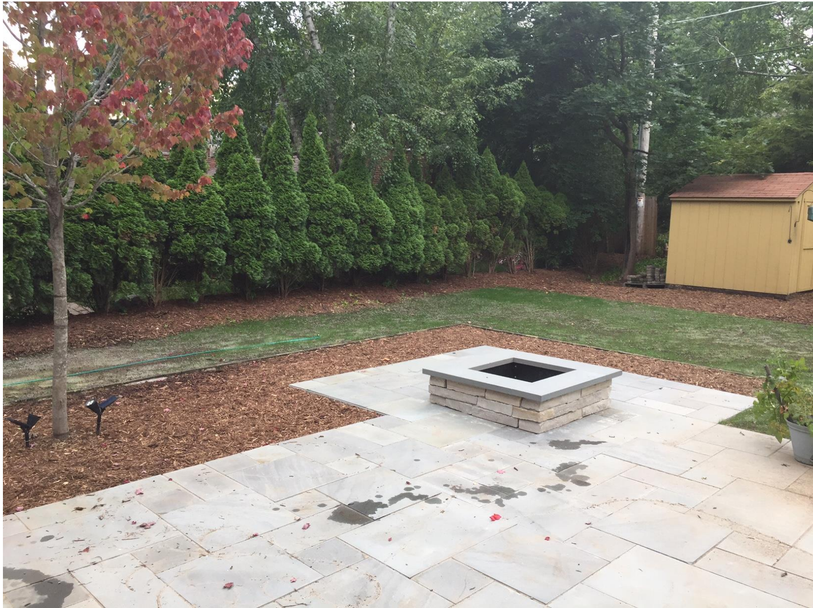
Partially completed work with firepit and new tree at left.
