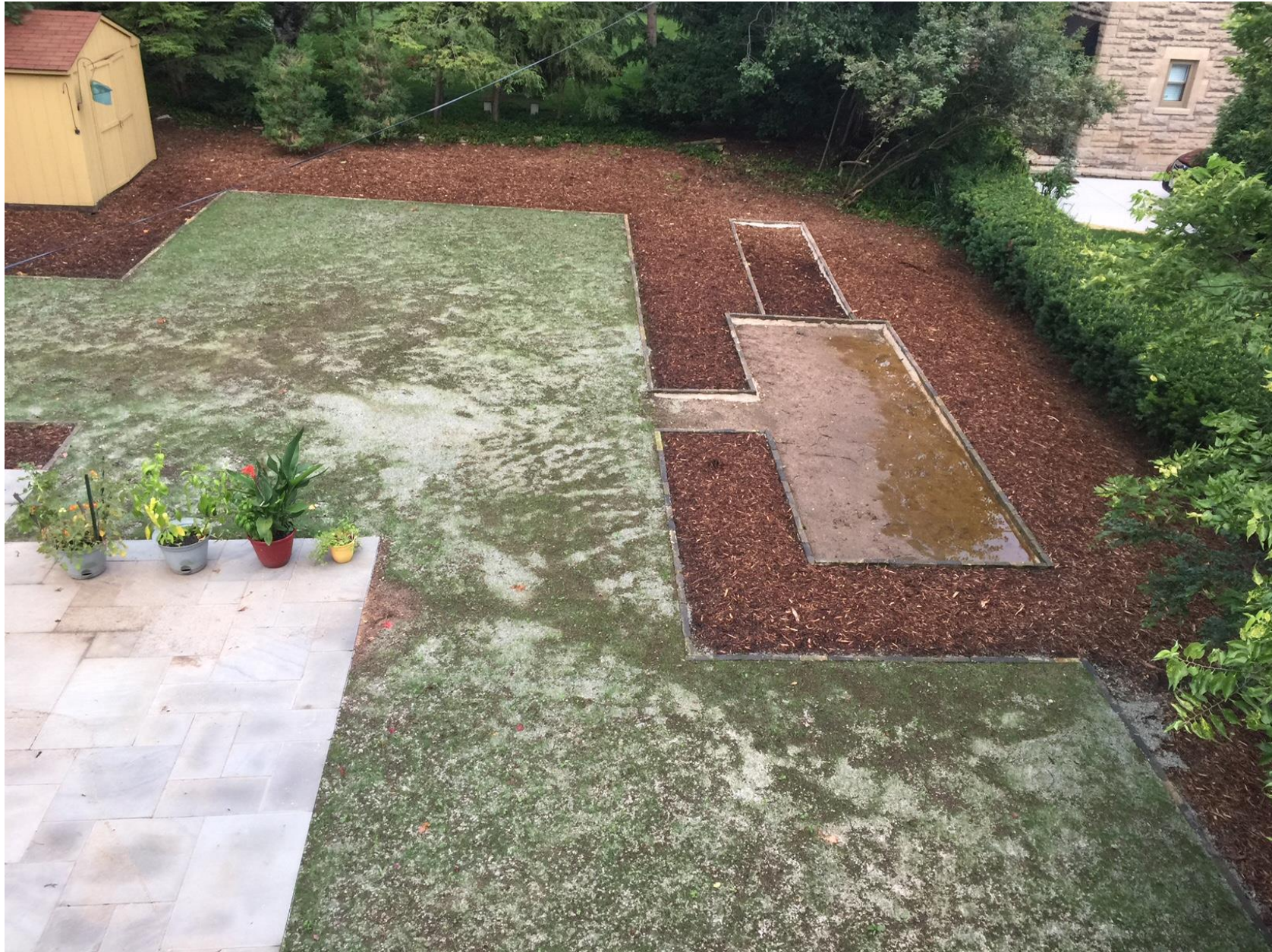
Partially completed work
