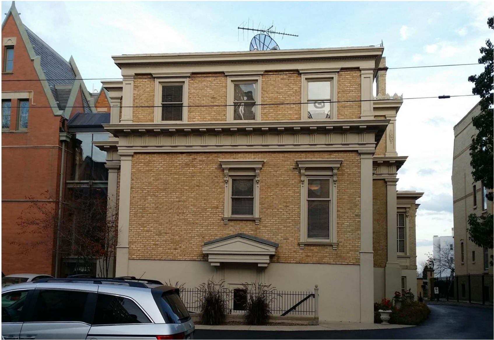
Windows in 1994 addition
