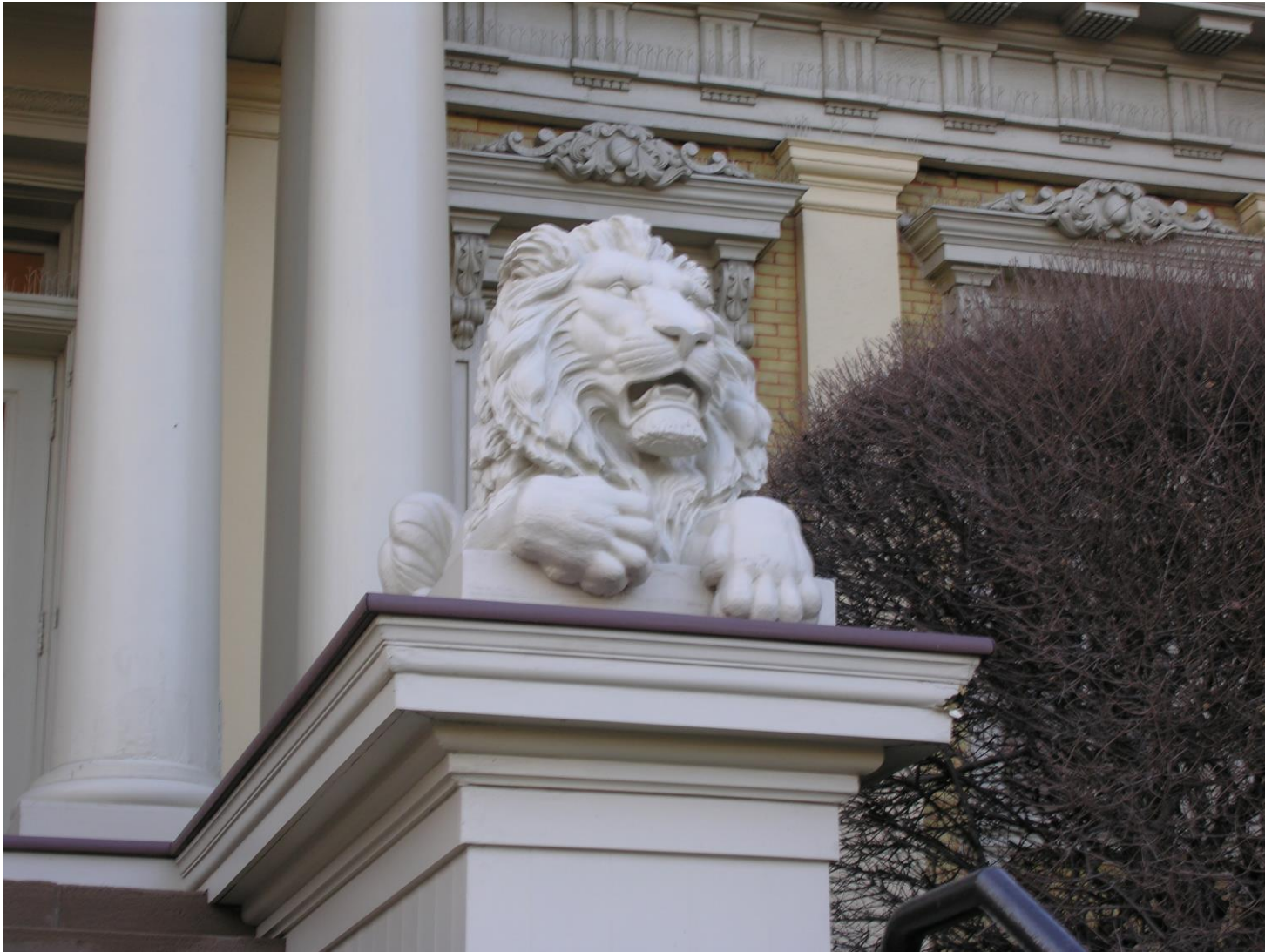
Repairs to statuary and pedestals
