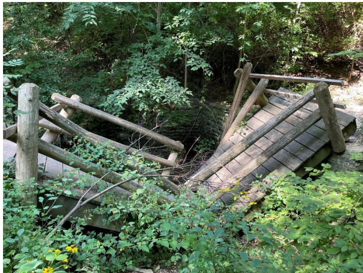
South Lighthouse Ravine bridge3
