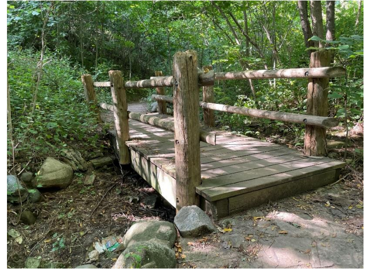
North Lighthouse Ravine bridge 803-2
