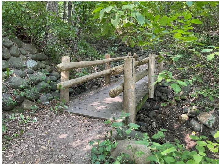
North Lighthouse Ravine bridge 802
