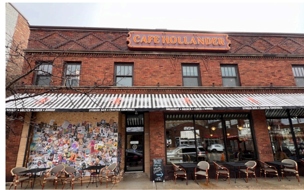
IMAGE #1 - EXISTING EXTERIOR
