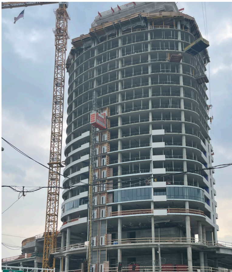
Work Progressing Summer 2023.
