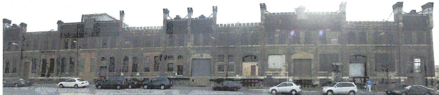
3 CURRENT CONDITION PHOTOGRAPH - FOR REFERENCE ONLY
