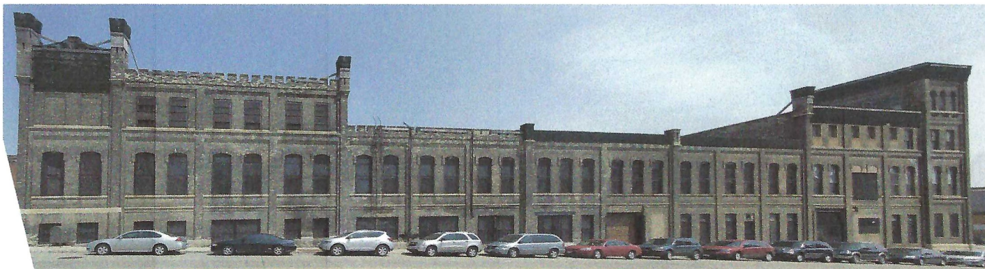
3 CURRENT CONDITION PHOTOGRAPH - FOR REFERENCE ONLY
