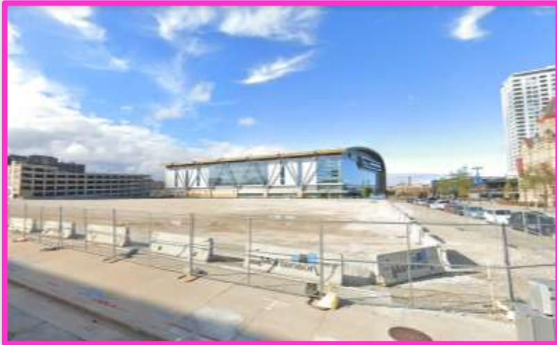
View from W State St looking north
