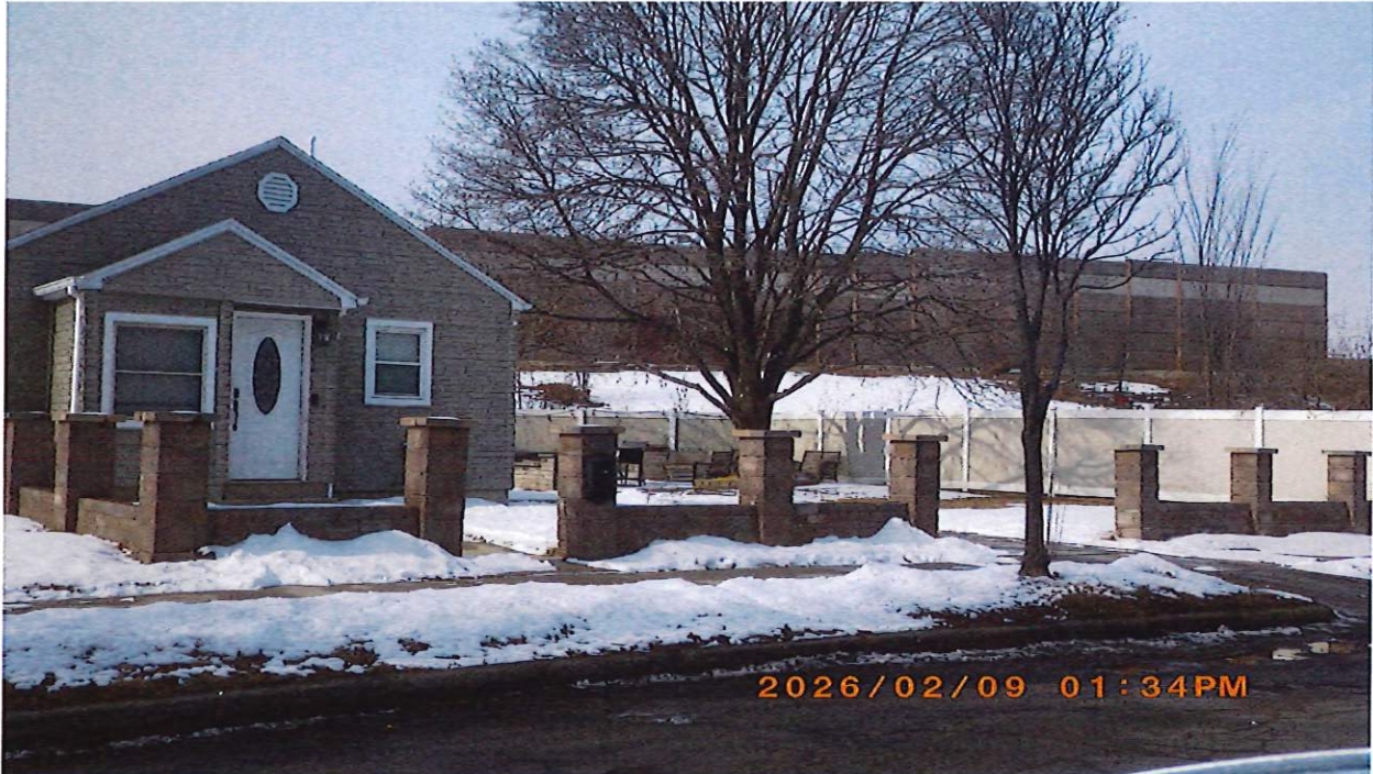
3263 S 3rd Street. (2/9/2026) (G. Armstrong/ Special Enforcement) (ORD-25-03604. Violation #1)
